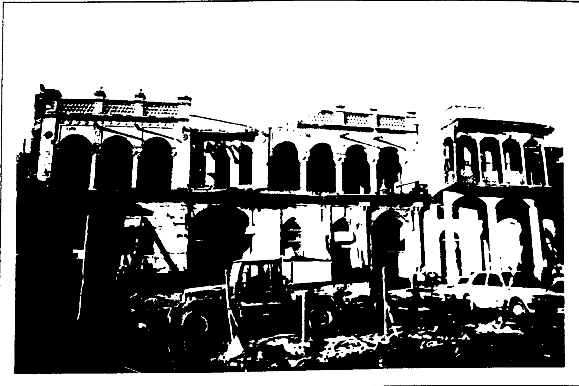
Figure [6-4] The devastation of the Corniche Area of Shatt-al-Arab, Basrah. [Source: The author, 1989 ]
