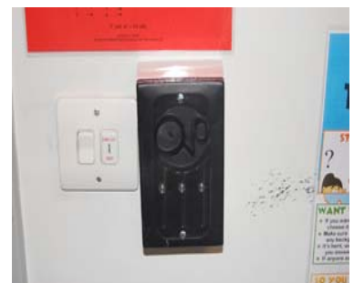
Fig.6.40. M:SD 2.0 P:3 CO 2 sensors
