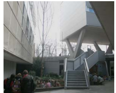
Fig.6.34. M: FP 0.0 P:19 V shaped columns in Fort Pienc
