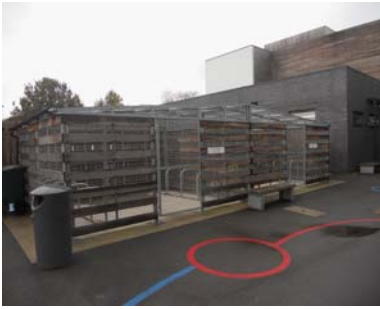
Fig. 6.47. M:SD 0.0 P:18 Safe bike storage in bike sheds in Silverdale school.
