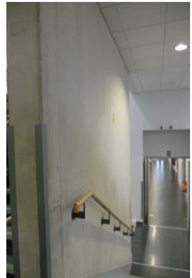
Fig.6.33. M: SD 1.0 P:14 Concrete walls
