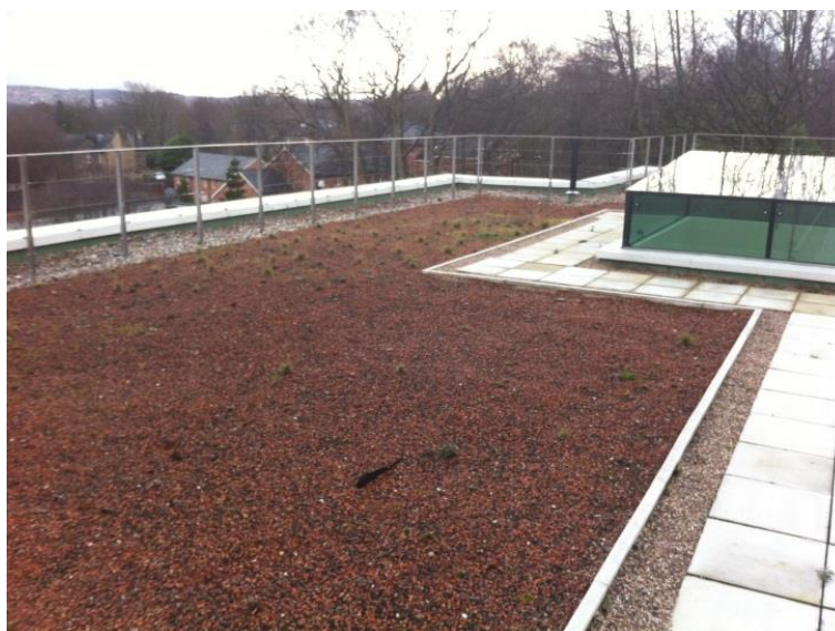
Fig. 2.1 Extensive green roof on top of a building at the University of Sheffield
