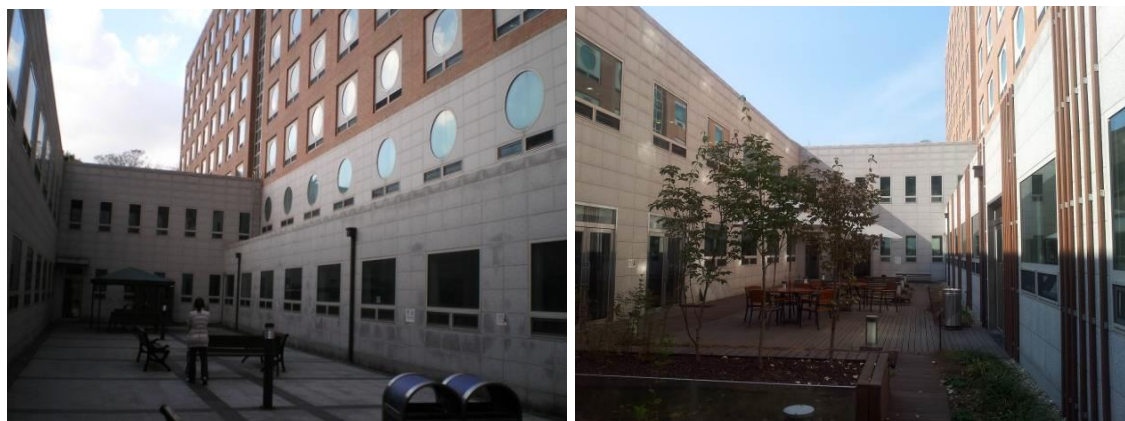
Fig. 6.1 Site conditions before (left) and after (right) the refurbishment using vegetation, wood decking and street furniture
