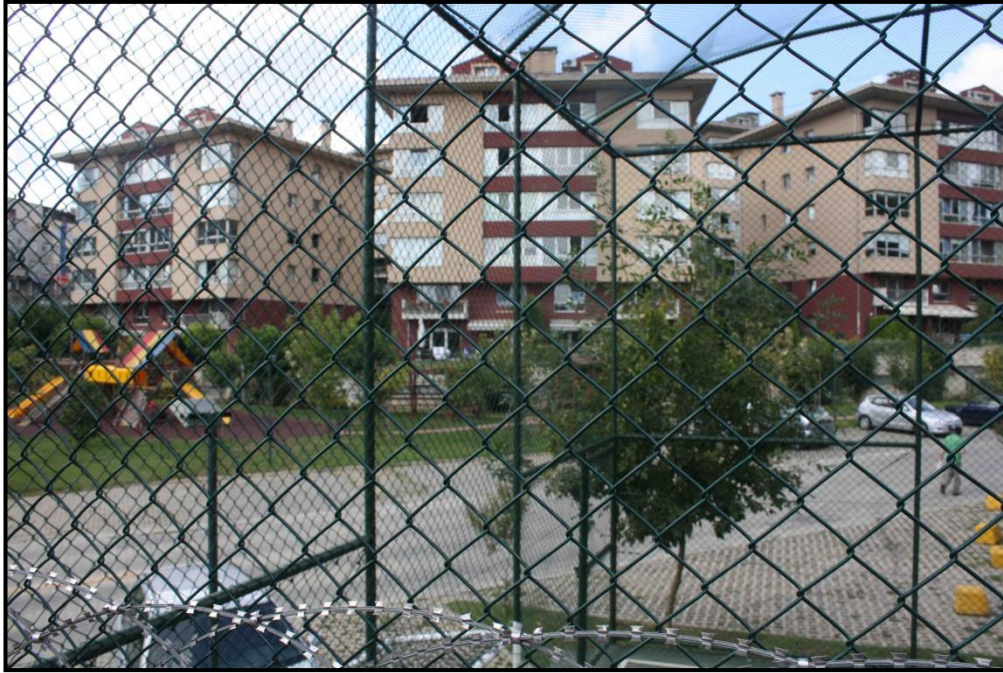
Photo 7.4: A view of MESA Houses behind the fences.
