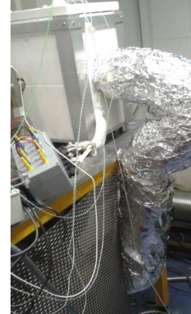
(c) Second layer of insulation with Aluminium foil over-wrap
