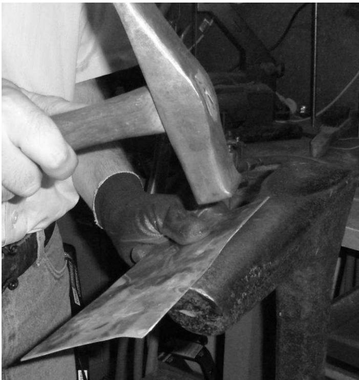
Figure 96. Curling from the exterior.
