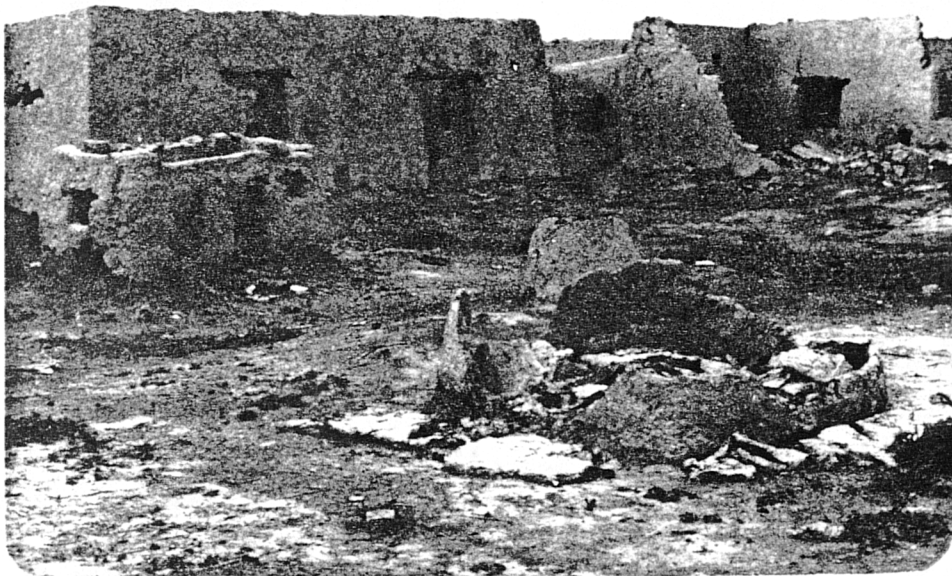
Plate 1-4 : A view of a damaged village
