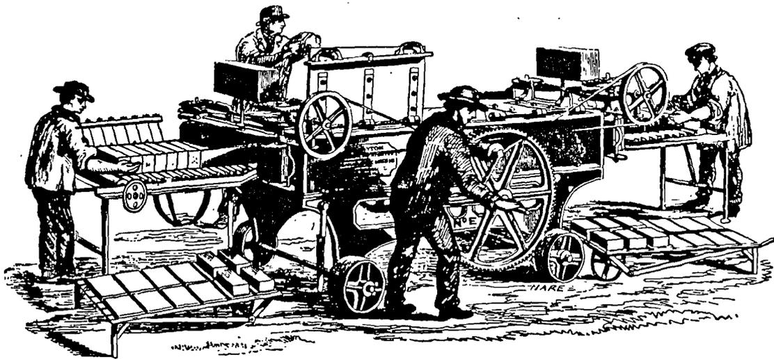
Figure 6.3. Clayton's "No. E" General Purpose Brick and Tile Machine.
