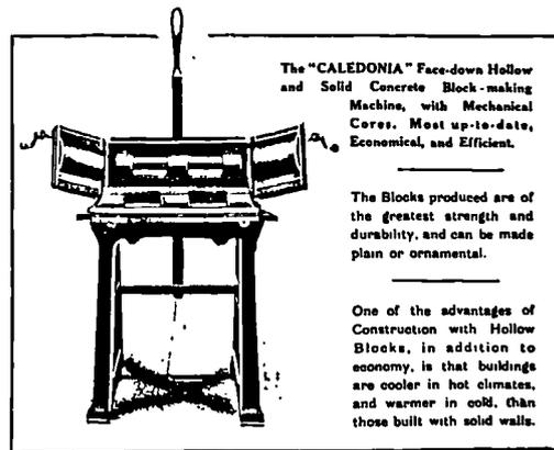
Figure 11.15. The "Caledonia" concrete block machine and moulds. [From The "Caledonia" Concrete Block Machine Company (n. d.) p. 4-5]
