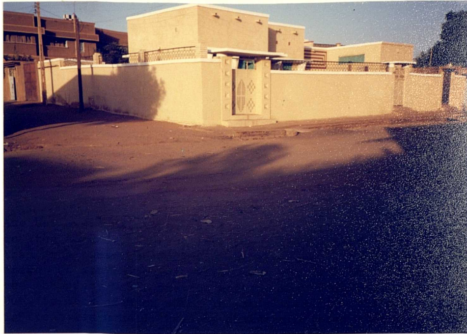
PLATE (6.16): Another well maintained single-floor courtyard dwelling in the Al-Umda Sharque locality, that looked smarter than the two-floor building at the rear with curtains drawn on its balconies. Also, see the two entrances of the boundary wall, one for men and the other for women. Due to lack of open space in this locality, the street in front was usually used by children to play football.
