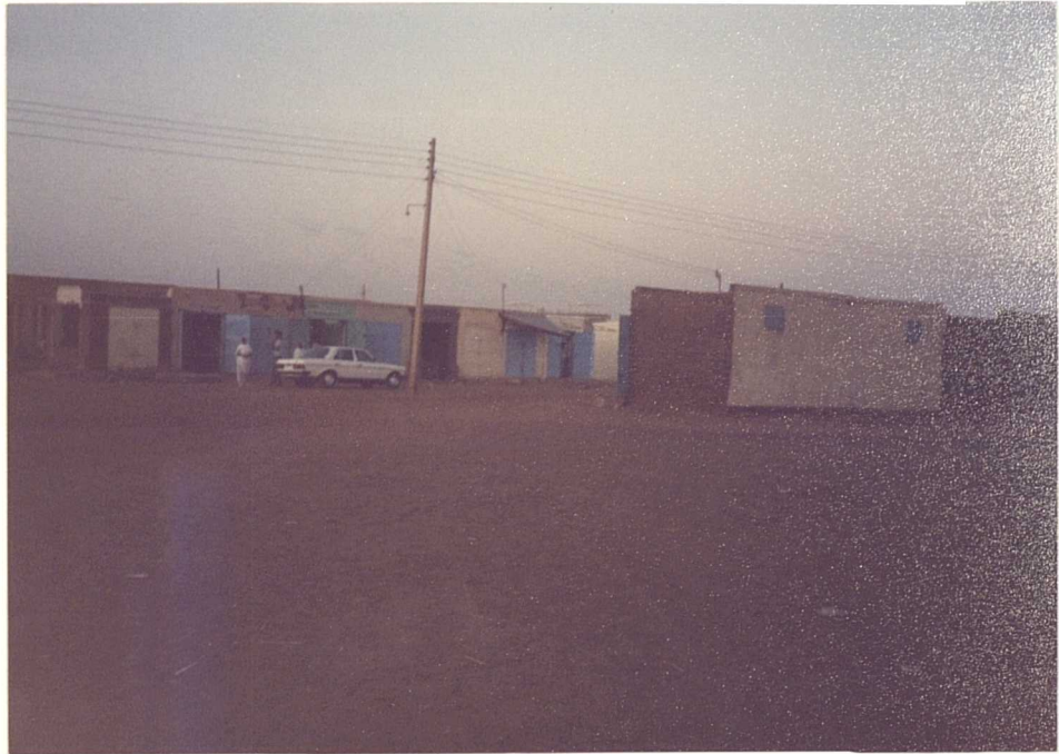
PLATE (6.22): The northern part of the Al-Mahadia Hara-2 central market with plenty of space in between.
