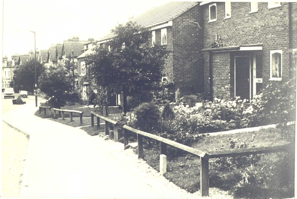
PLATE (8.12): The low wooden fence, texture added by hard surfaces and plants and colours all are personalization features for the front gardens.. Terrace housing, York U.K.. (Photograph by the author).
