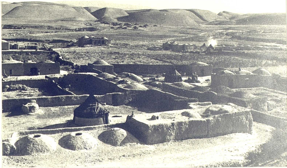
PLATE (4.3): An Afghan village consists of houses with domed mud-brick chambers grouped around courtyards, in which are pitched the tents of nomadic relatives, constructed of felts tied around collapsible wooden frames. The same form of tents can be made of thatch indicating that buildings made of different materials can take similar forms (after Grube, E. J., Architecture of the Islamic World ).
