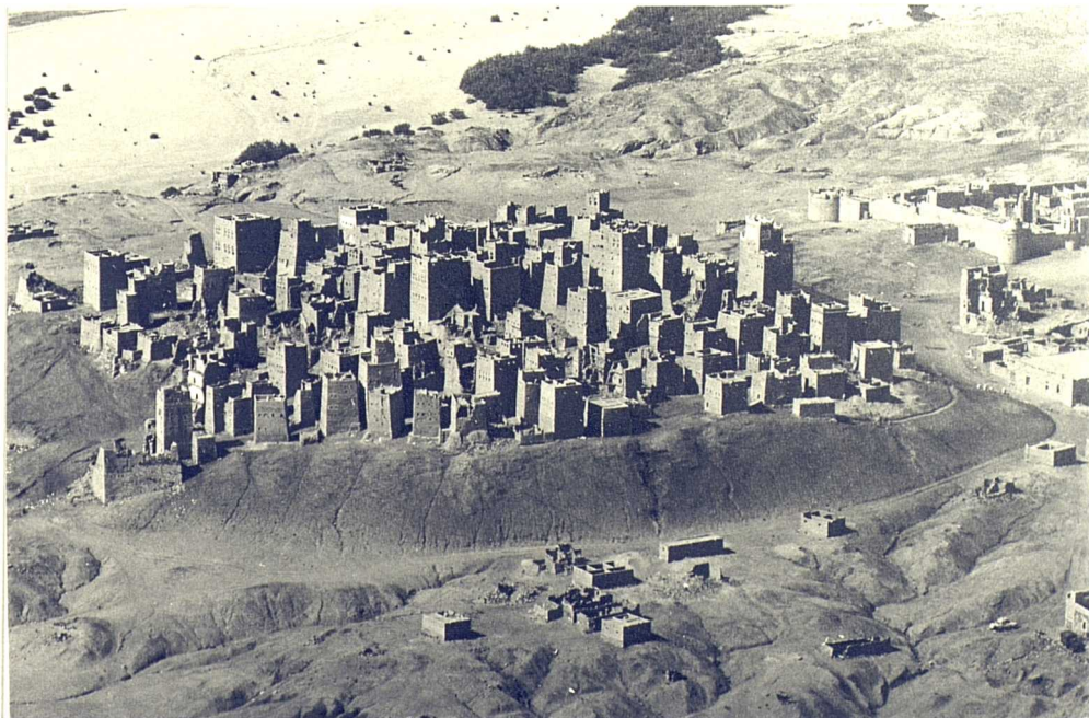
PLATE (4.6): Tower-houses are characteristic of the uplands of the western Arabian peninsula, such as these in the city of Marib, central Yemen. The settlement is unprotected by walls, "each" house becoming a "fortress" in times of trouble (after Grube, E. J., Architecture of the Islamic World).
