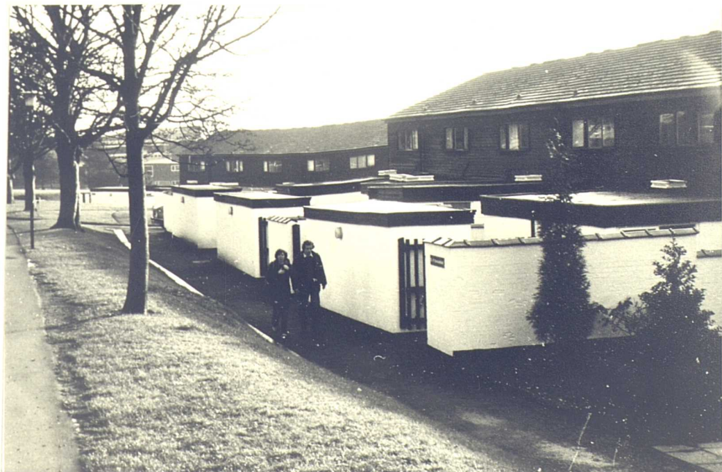
PLATE (8.5): Solid walls are the common territory controller. They provide visual and, if of adequate mass, acoustical privacy. Student hostel, University of York, U.K.. (Photograph by the author).
