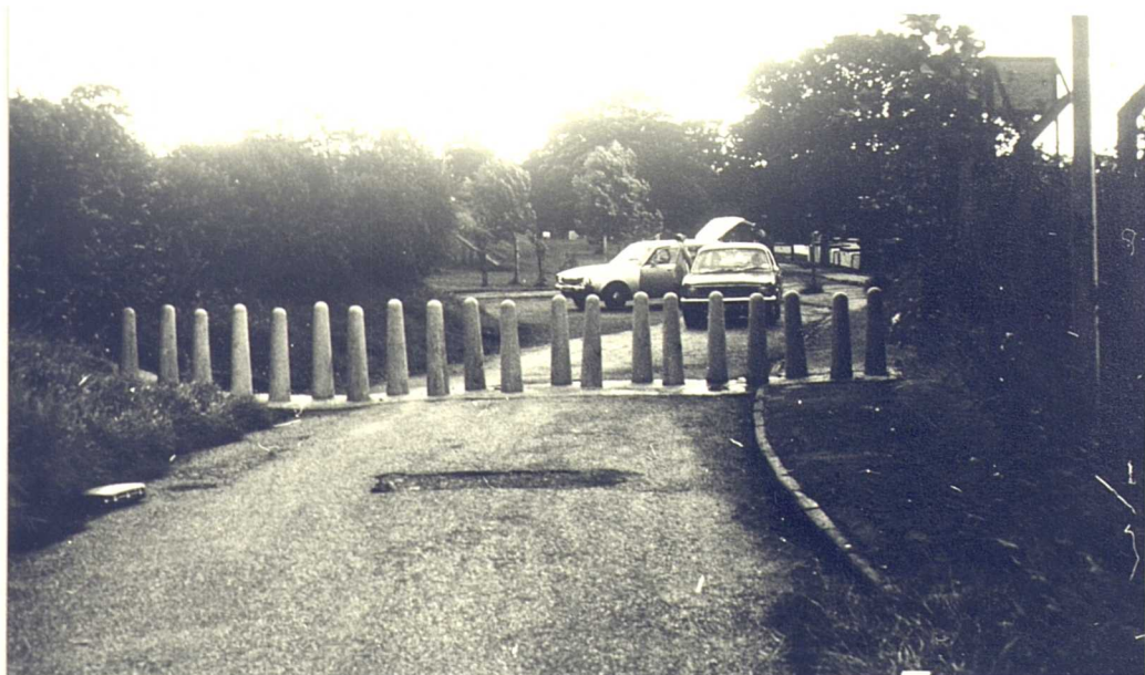
PLATE (8.11): An effective circulation 'filter'. The concrete posts has been made to replace a solid wall to allow visual surveillance for safety reasons, York, U.K.. (Photograph by the author).
