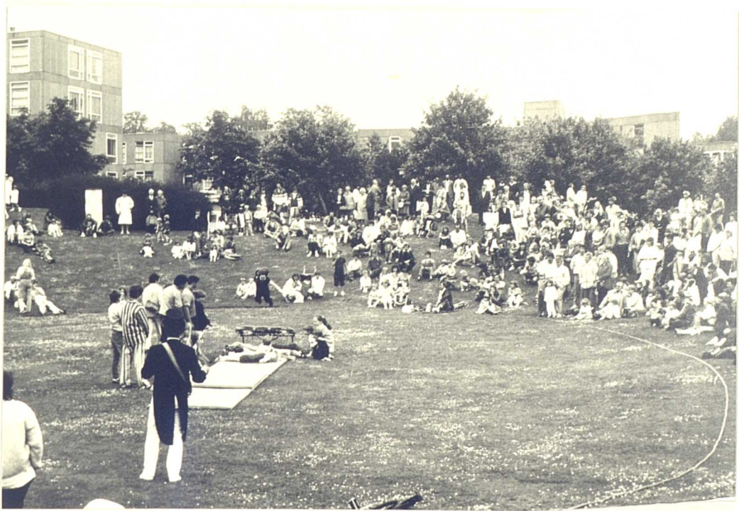
PLATE (8.16): The proper use of planting can provide a sense of containment, visual and acoustical privacy. Here the plantain screens off the public from the students hostels, amphitheatre at the University of York, U.K.. (Photograph by the author).
