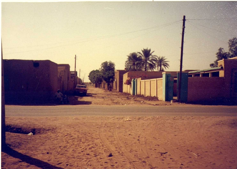
PLATE (6.17): Eddoma asphalted road and a street running north south in Al-Umda Sharque. See the two green entrances, one for men and the other for women, representing the effect privacy. Also, note the tiny high level window of the kitchen, to the left facing the road, where extreme privacy was needed in such space.
