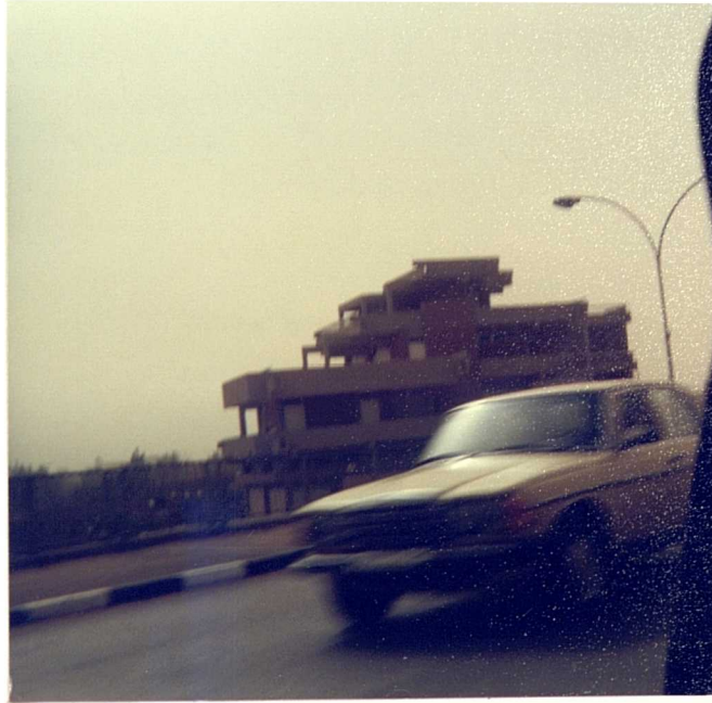
PLATE (7.4): The tradition towards staggering balconies and roof terraces, with their low walls, subject the building to a greater degree of visual privacy loss and exposure to sun rays during the day.
