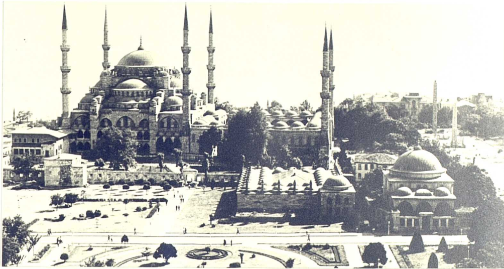
PLATE (4.7): The mosque of Sultan Ahmed in Stanbul. It is covered by a dome and buttressed by semi-domes and has six minarets (after Grube, E. J., Architecture of the Islamic World).
