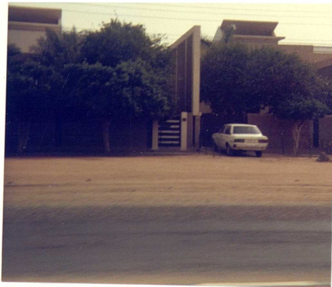
PLATE (7.5): Can the poor afford to build a party-wall as high as this to prevent being overlooked by the rich?!
