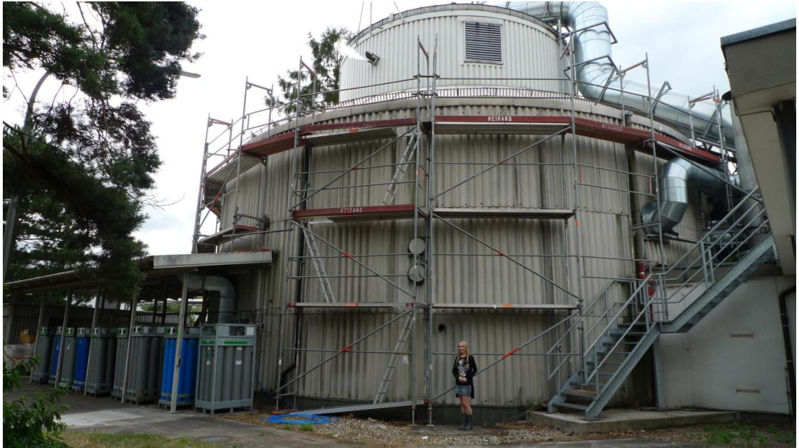
TLM in front of the AIDA facility.
