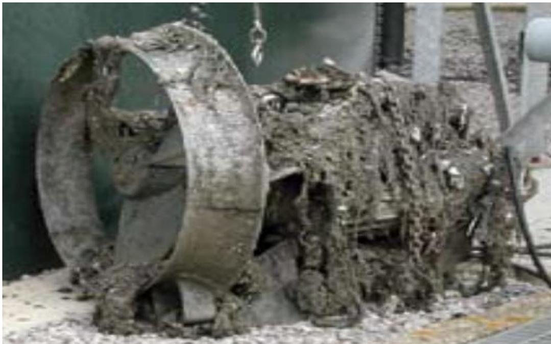
Figure 2.7: Submersible mixer is lifted out from the digester for cleaning
