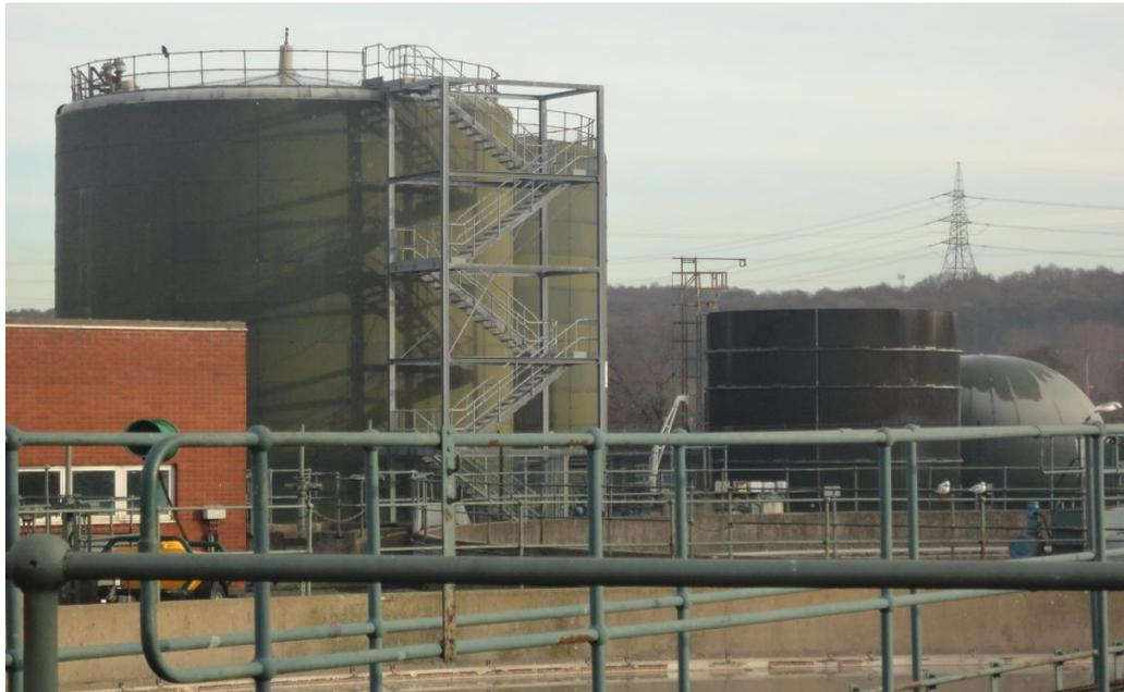
Figure 2.3: Mesophilic anaerobic digesters located in Woodhouse wastewater treatment plant in Sheffield, UK
