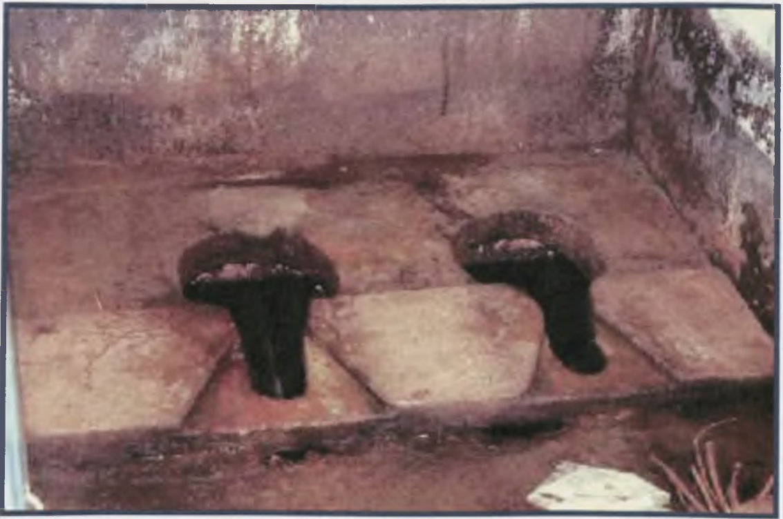
Plate 9 Squat hole arrangement in the KVIP
