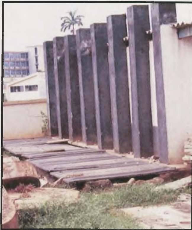
Plate 8 A public toilet: multiple pit VIP latrine locally called the KVIP
