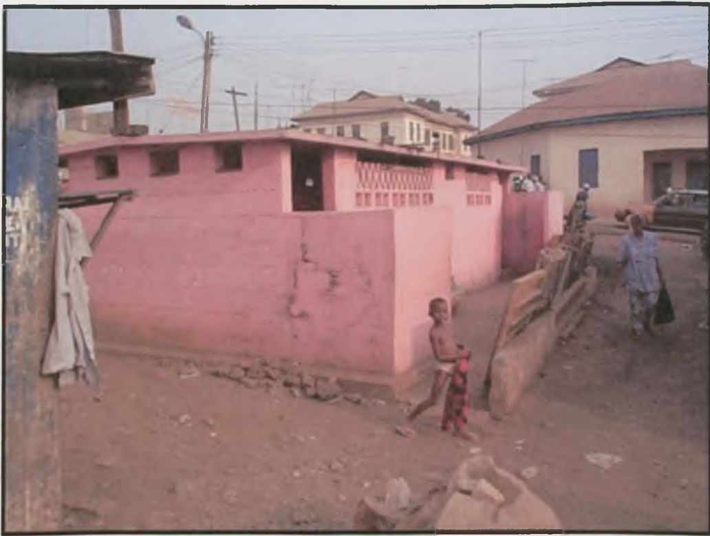
Plate 5 A public toilet: non-flush aqua privy
