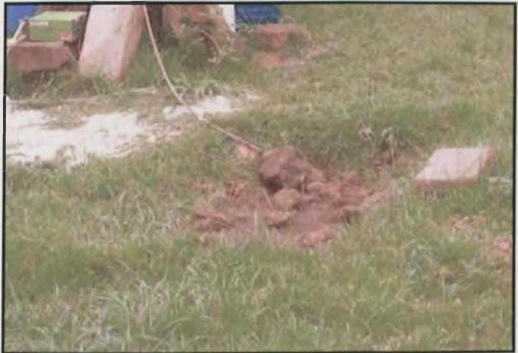
Plate 32 Pit filled with stones – receives effluent from reactor
