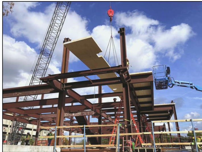
Figure 1.1: Hybrid steel frame structure with CLT floors under construction (Source: AISC, 2022)
