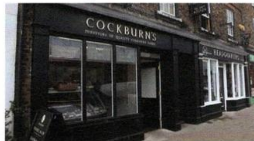
Shops in Bedale after the newly reinstated shop front
