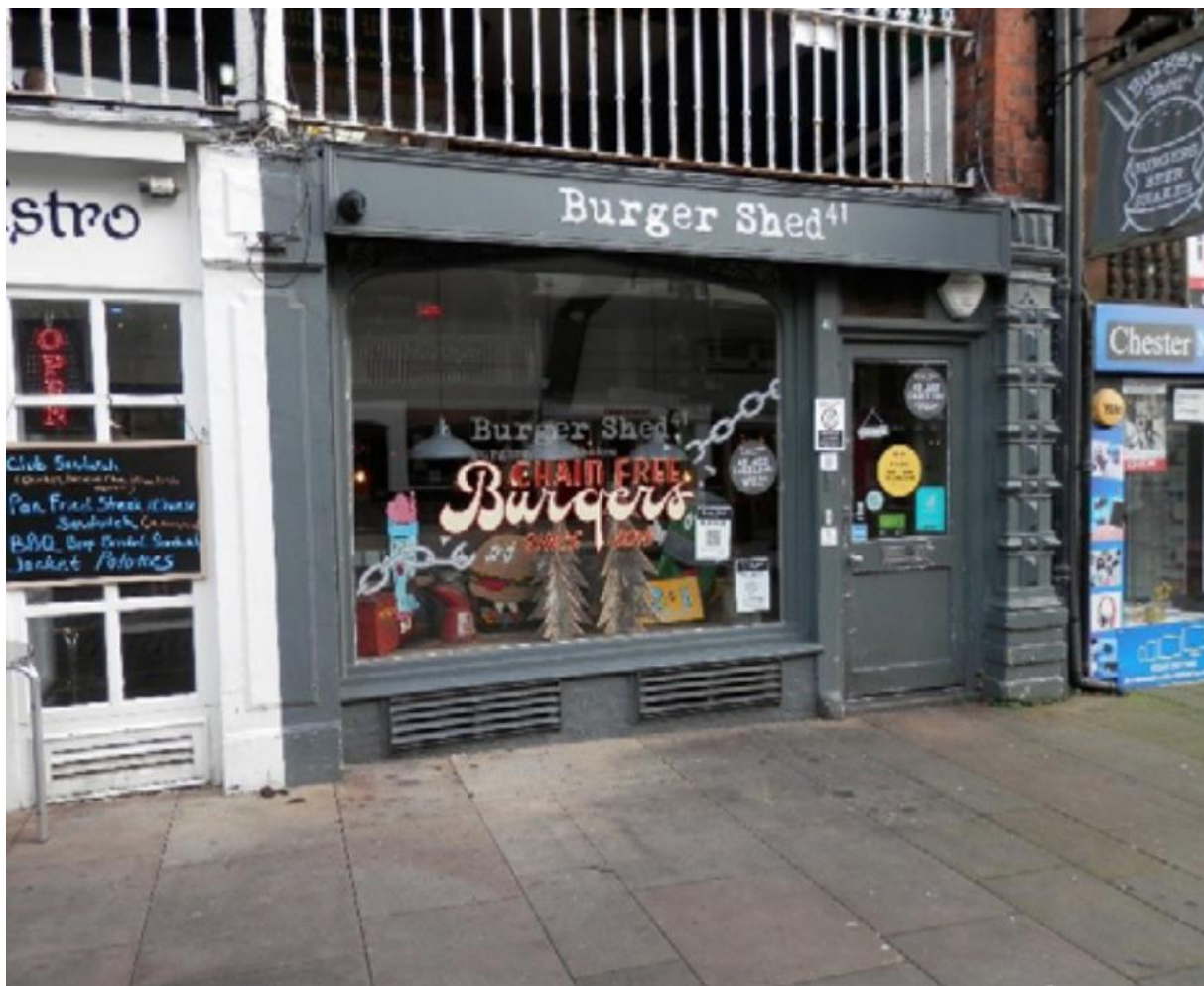
Figure 87, an example of an improved shop front façade (Donald Insall 2022b).
