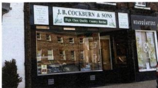
Shops in Bedale before reinstatement
