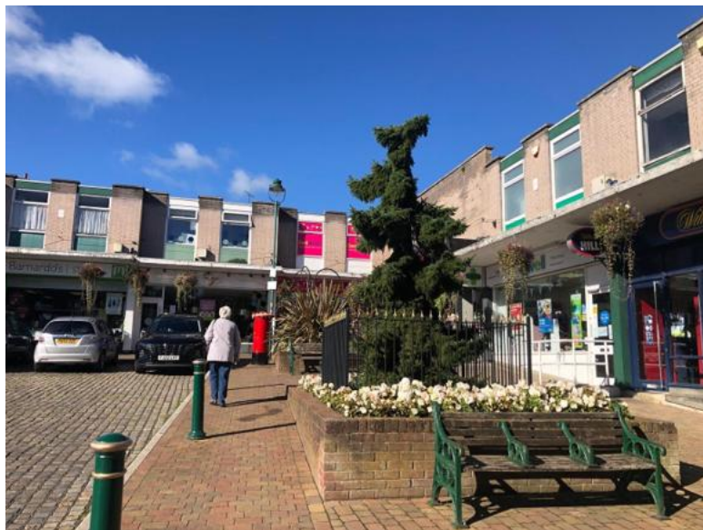
Figure 73, the 60's buildings around the Market Square.
