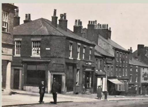
Fig. 3 - The building that was demolished to make way for the bank building.
