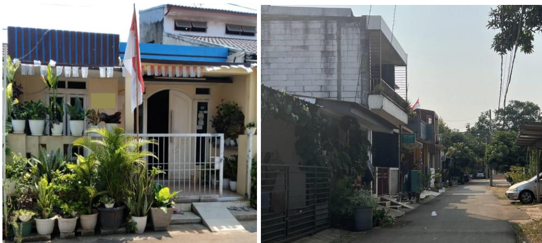
Figure 4.16 A Type 21/60 home after renovation (left) and its surroundings (right)
