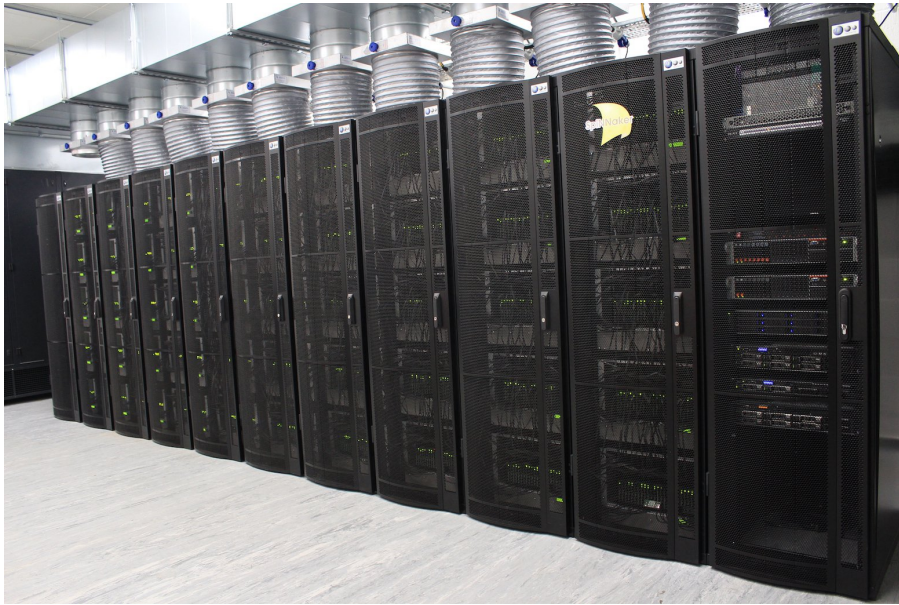
Figure 1.17: The SpiNNaker Project
