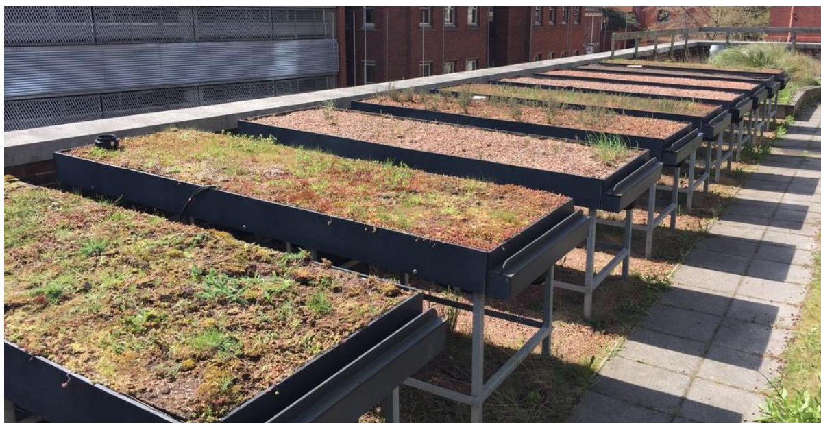
Figure 2.3. University of Sheffield green roof performance monitoring test bed, during vegetation establishment phase
