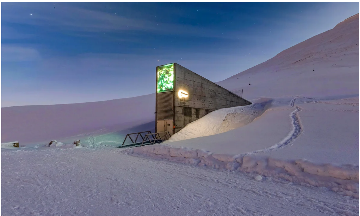
FIG 3.2. External view of the Svalbard Global Seed Vault.
