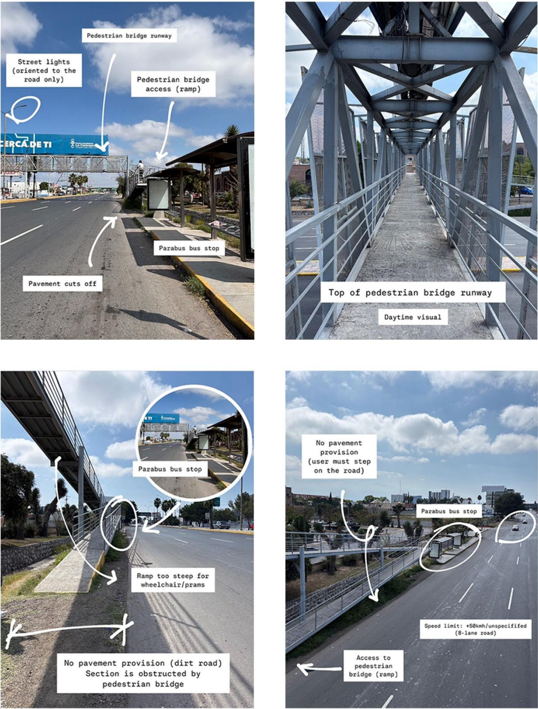
Figure 7: Visual analysis of a bus stop next to pedestrian bridge in Saltillo, Mexico
