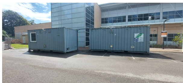
(a) The DOMESTIC facility, exterior
