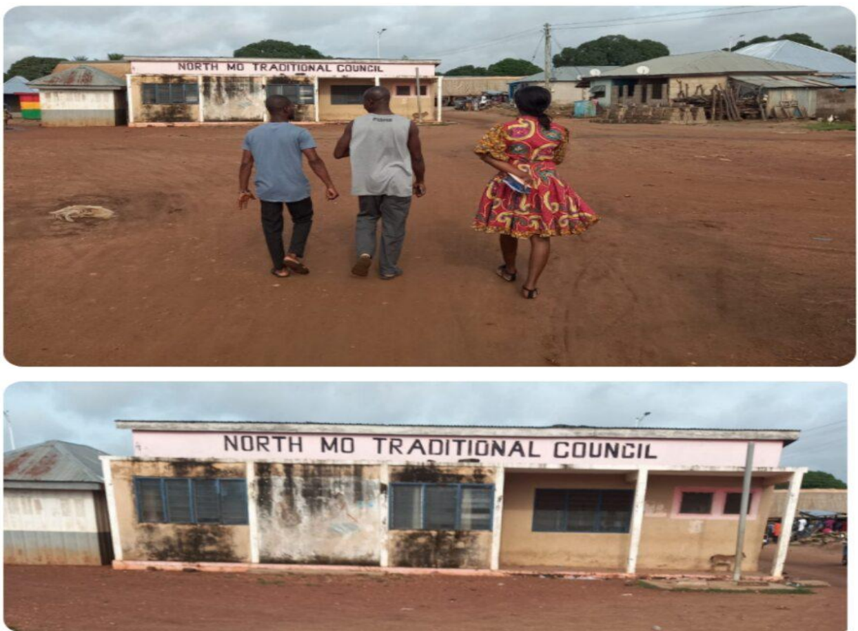
Figure 24: North Mo Traditional Council’s Office – Bamboi
