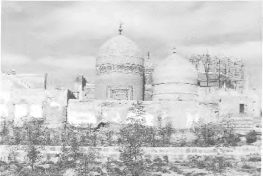
Figure 6.2 Photograph of the shrine at Ardabil reproduced from [Canby, 1999, p. 11]
