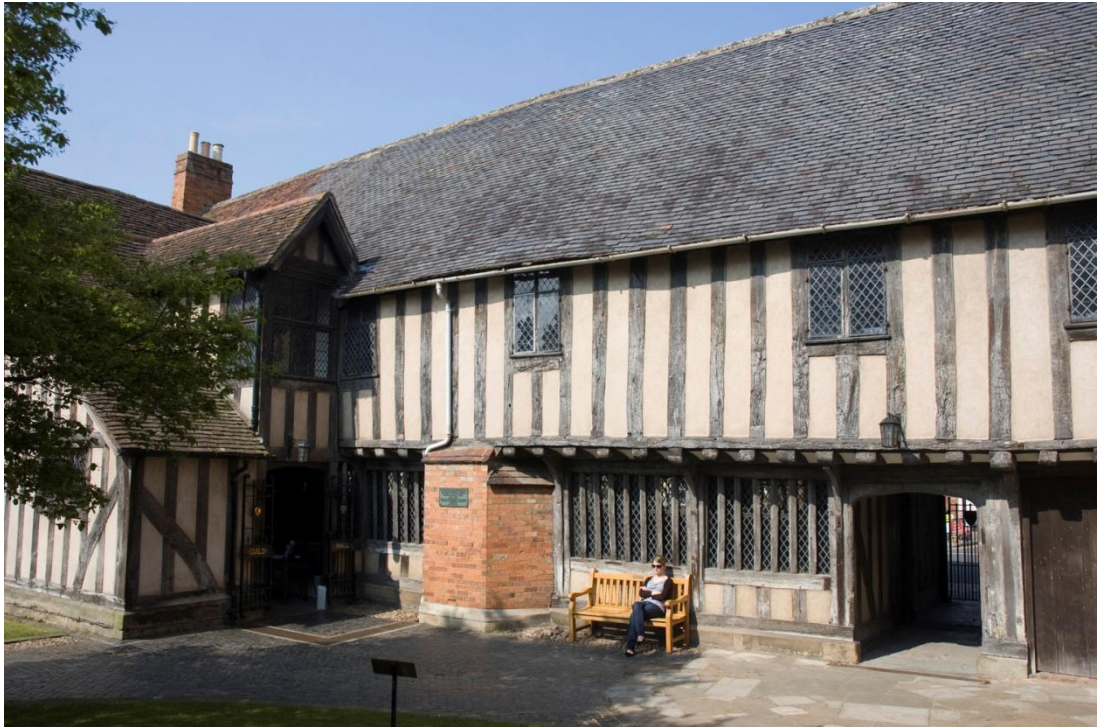
Figure 7 – The Guildhall, east elevation
