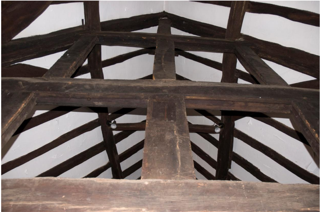
Figure 11 – Trusses showing grooves for infill panels.
