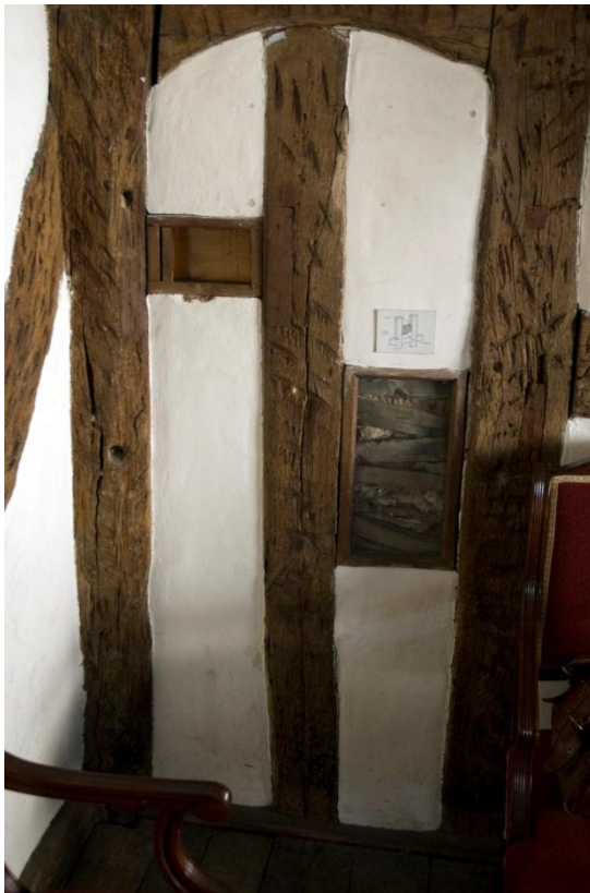
Figure 10 – The blocked door to the 'prevey'
