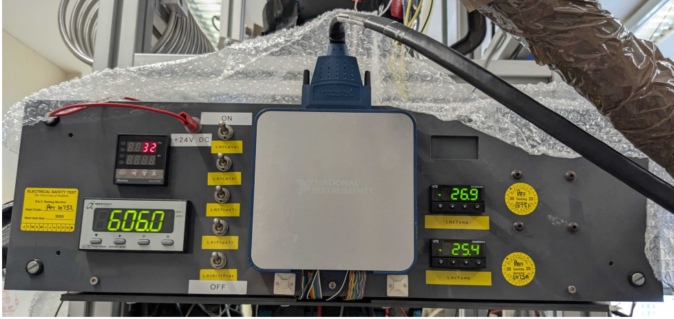
Figure 8.8: Live tracking of thermal parameters such as LAr/LN temperatures and pressures, as well as the argon liquid level on a NI PXI-6229 slow DAQ live monitor system. Pictured displaying relevant parameters for a dewar filled with air.
