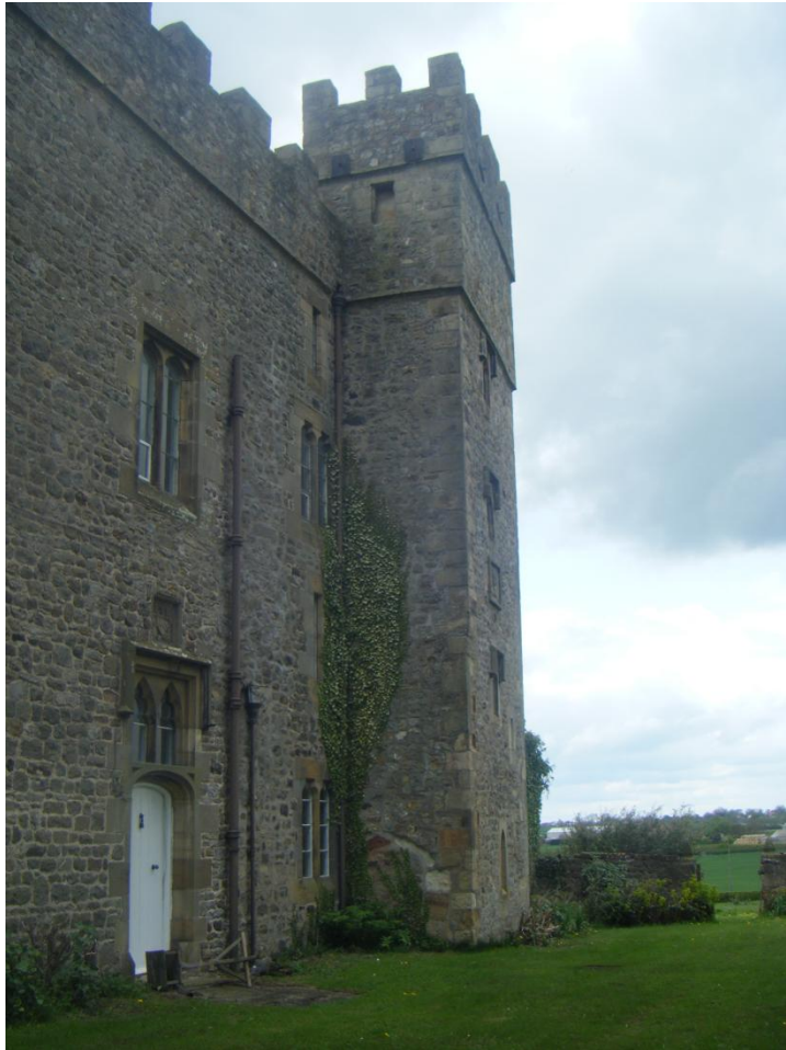
Figure 27 The eastern turret, Cowton Castle. Stairs, accommodation and privies were located within the two turrets, late 15 th century.
