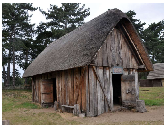
Figure 2.2.2: A post built house at the West Stow visitor centre. (St Edmundsbury Chronicle, 2009).
