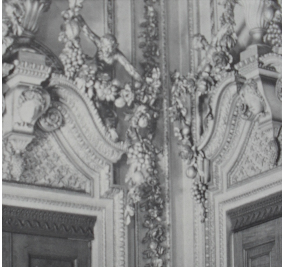
Fig. 35. The Embellished Doorframes at Norfolk House, photographed before demolition in 1937.
