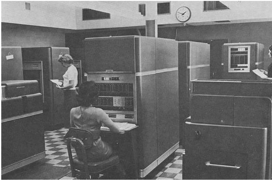
FIGURE 1.1. The IBM 650 Magnetic Drum Calculating Machine, created in 1953. The machine is considered to be the world's first commercial computer to generate any meaningful profit. Output was presented using a display panel of bi-quinary light indicators. Long term memory storage was provided by the IBM 727 Magnetic Tape Unit, while short term memory was stored using the magnetic drums. Magnetic core memory was also used, as part of the IBM 653 High-Speed Storage Unit. (Image: IBM Archives).
