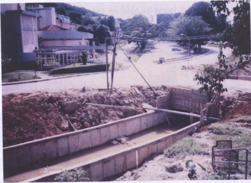
Figure 5.4b. Part of the Pantai River from which natural protection was removed and concrete slabs installed in 1998.
