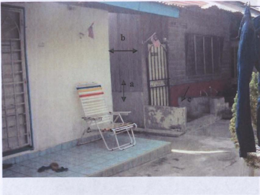
Figure 7.2. A typical house in Kampung Haji Abdullah Hukom. Note the mix of bricks and wood (see arrow a), the distance between the two houses (arrow b) and the protection against flooding in front one of the houses (arrow c).
