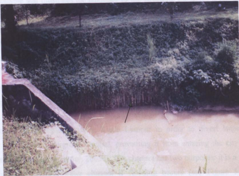
Figure 5.4a. A part of the Pantai River on which natural protection in the form of a barrier of branches was installed to control river bank erosion before 1998 (see arrow).
