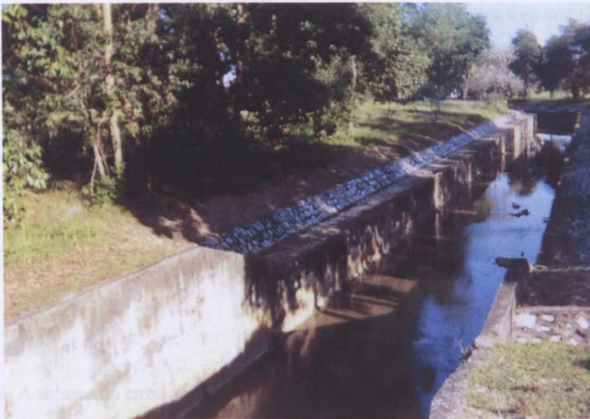
Figure 6.5b. A monsoon drain constructed in a residential area of Section 10, Shah Alam showing the correct size for monsoon drains.
