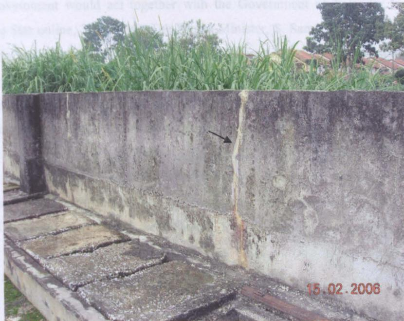
Figure 6.16. One of the cracks on the flood wall (see arrow).
