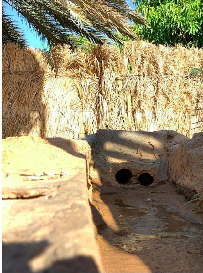
Photo 3.6: Clay pipes are used to get water from the well, then channels are used to disperse the water in Saudi Arabia (Mardhi Alenazy, 2020).
