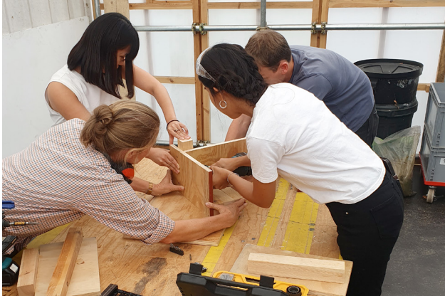
Figure 52 - Co-making the formwork
