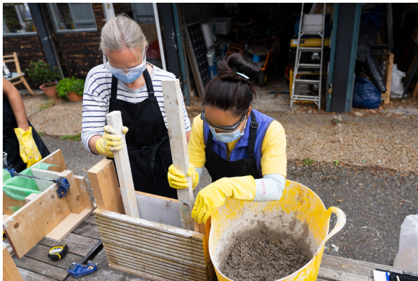
Figure 53 - Mixing and tamping the hempcrete mix
