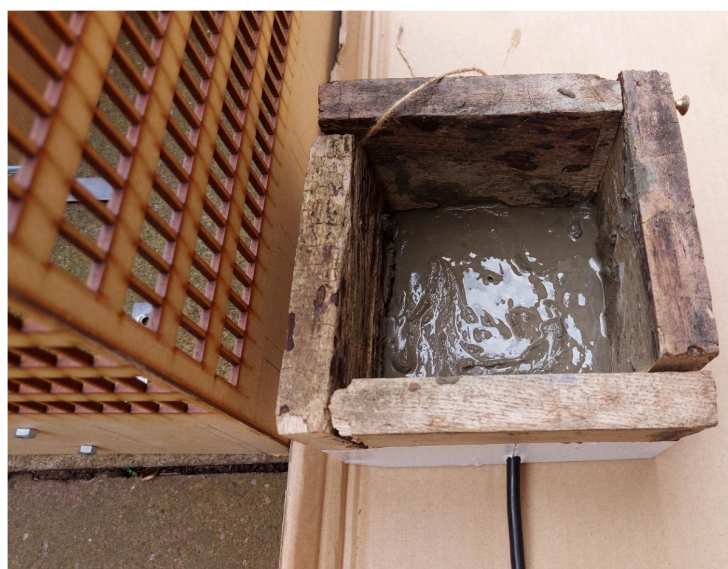
Figure 43: Casting of Pool
