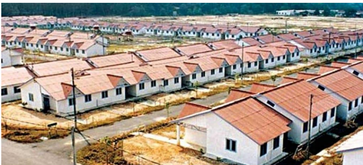
Figure 7 Showing estate layout without considering pedestrian walkway
