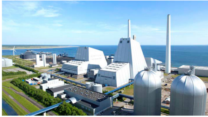
Figure 2.1 Avedøre power station, Denmark (Orsted, 2024)
