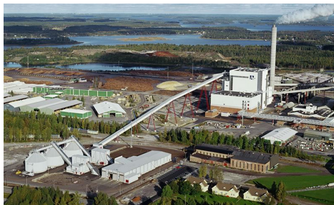
Figure 2.4 Alholmens Kraft power station, Finland (Alholmens, 2001)
