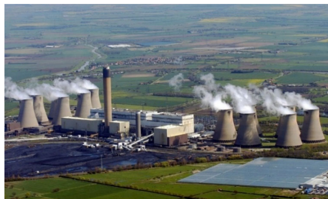
Figure 2.2 Drax Power Station, UK (YorkPress, 2014)
