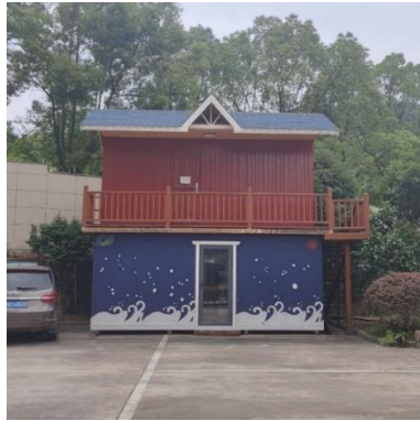
(a) CLT building
