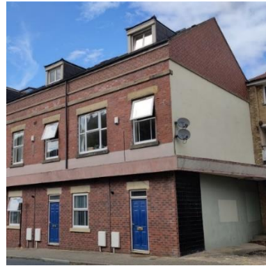
(b) Masonry building
