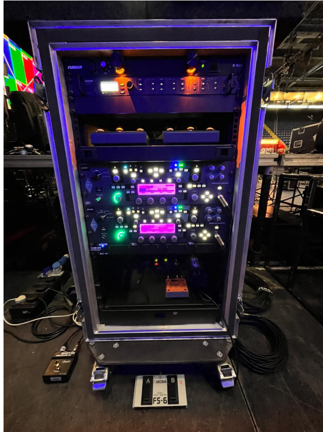
Figure 3: The rack in the picture demonstrates guitarist James Bourne of the band Busted’s Kemper and Spare Kemper unit (the units with the pink and green lights) in use during a soundcheck at the Nottingham Motorpoint Arena. The rack is positioned on a separate riser off stage, allowing the guitar technician to be in control out of sight of the performance area. Photo courtesy of Jack Mackrill.
