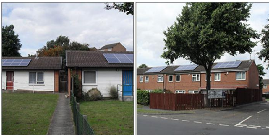
Figure 6.14 Meadows housing after PV installation (MOZES, 2012e)
