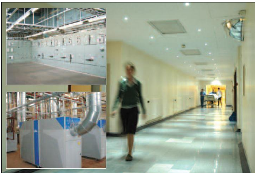
Figure 6.15 Examples of the energy efficiency lighting and boilers installed at Gwent Healthcare NHS Trust (Brind, 2008)
