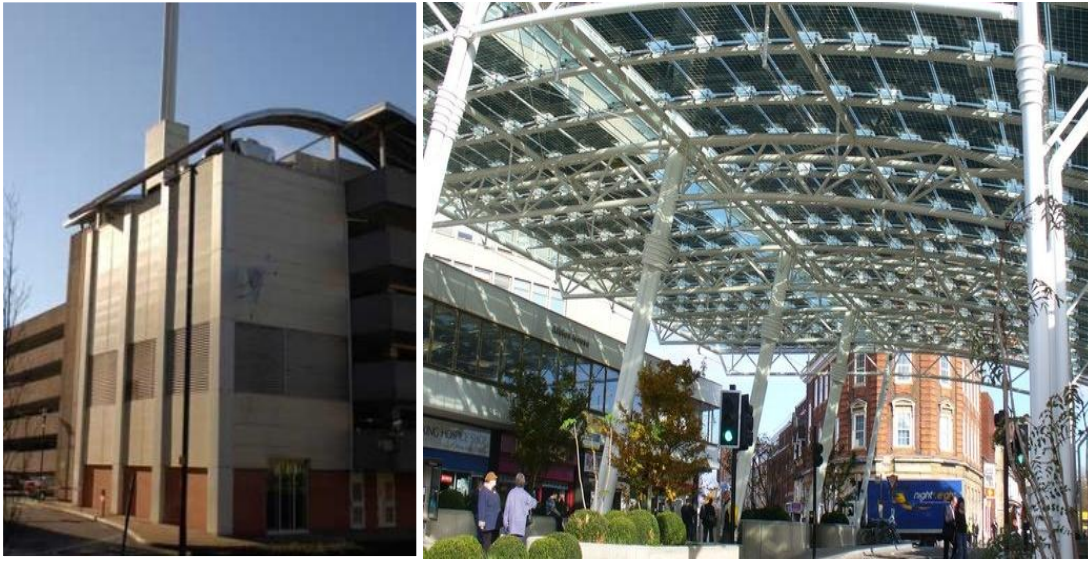
Figure 6.11 Woking town centre CHP plant (WBC, 2007c)
