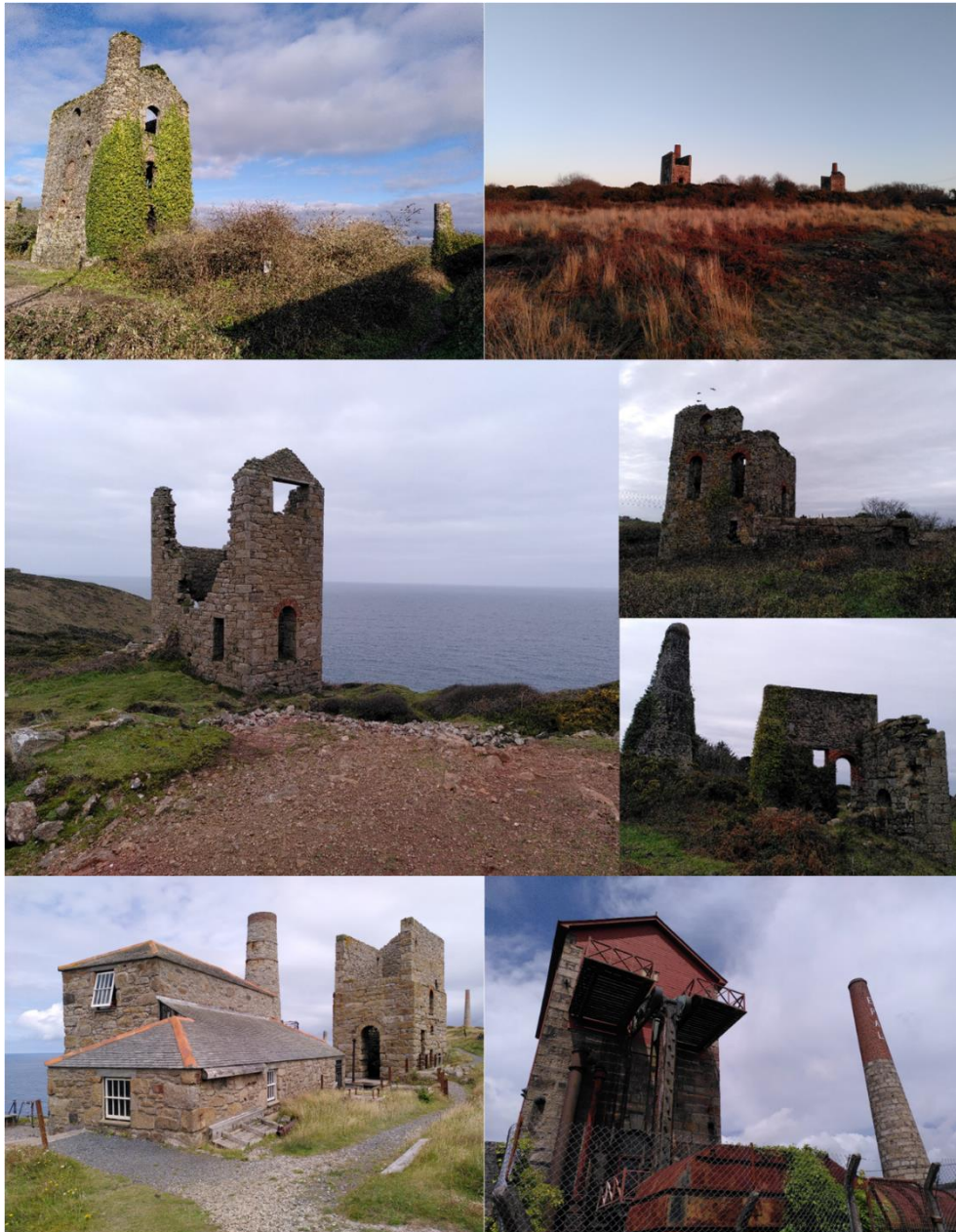
Figure 7.5: Cornish engine houses
