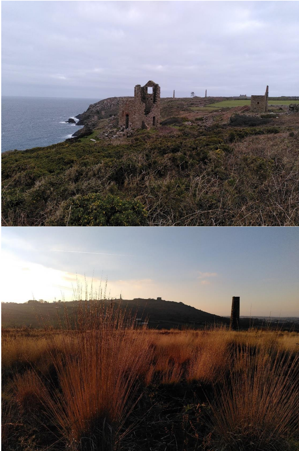
Figure 1.6: Remnants of the St Just mining district, looking north-east from Wheal Edward (above), and Wheal Uny, looking north-west towards Carn Brea (below). The hard, mineral-rich granite produced the Cornish mining industry, and the sea facilitated easy travel to mining districts around the world – with some interesting consequences for hookworm, as I will show. The Redruth-Camborne mining district clustered around the base of Carn Brae. 97 I will show that the existence of such a dense mining landscape shaped hookworm in particular ways.
