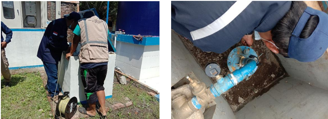
Figure 3.14 Pumping test and groundwater level measurement activities during fieldwork
