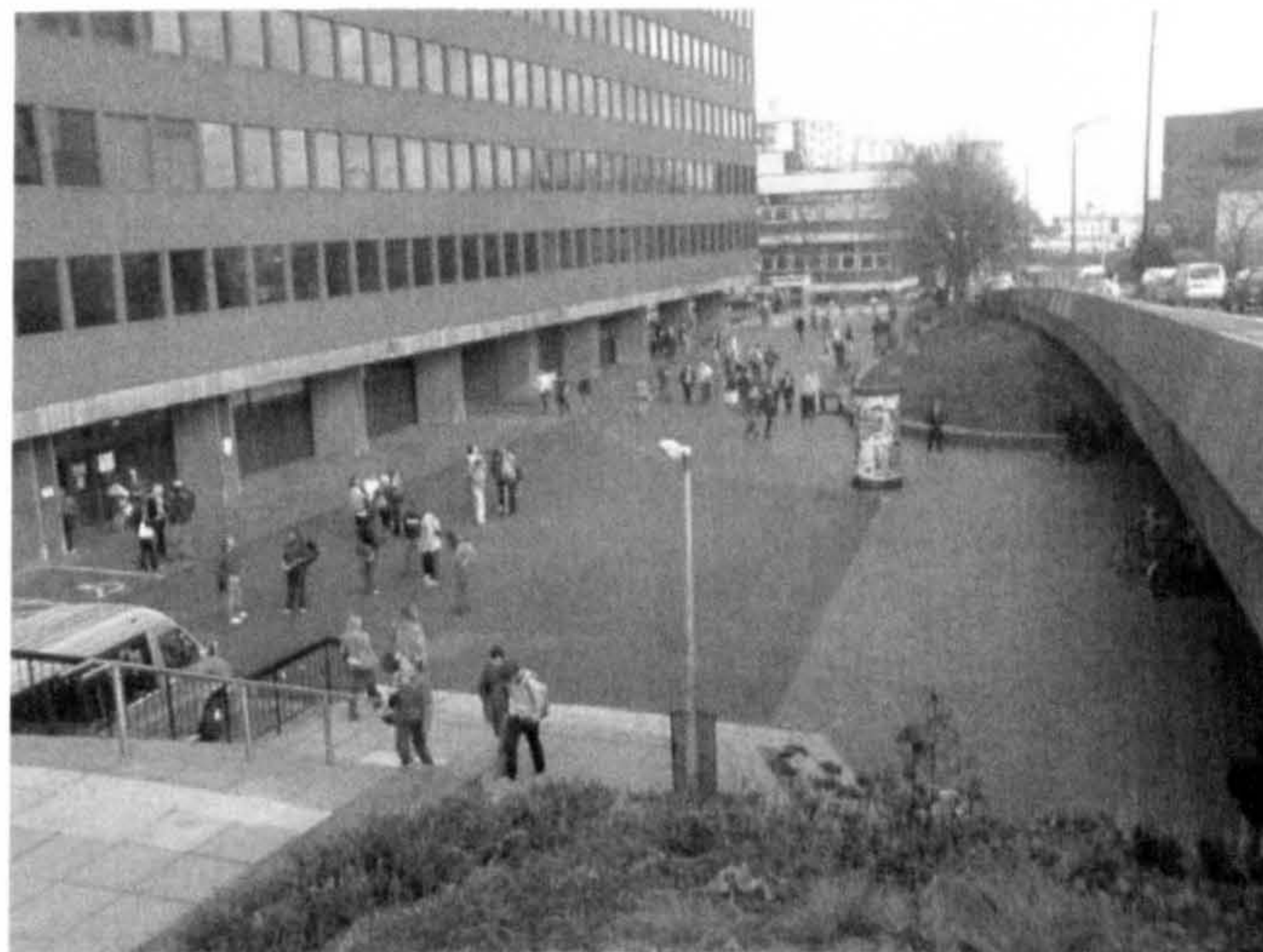
Figure 50: Alfred Denny Building and surroundings.
