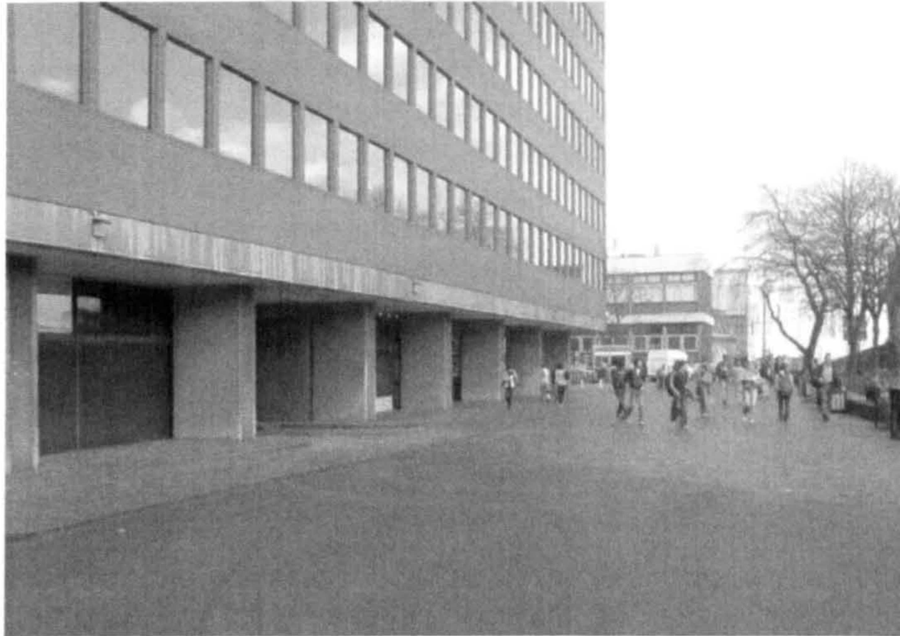
Figure 56: The façade of the Alfred Denney building and its pedestrian area.
