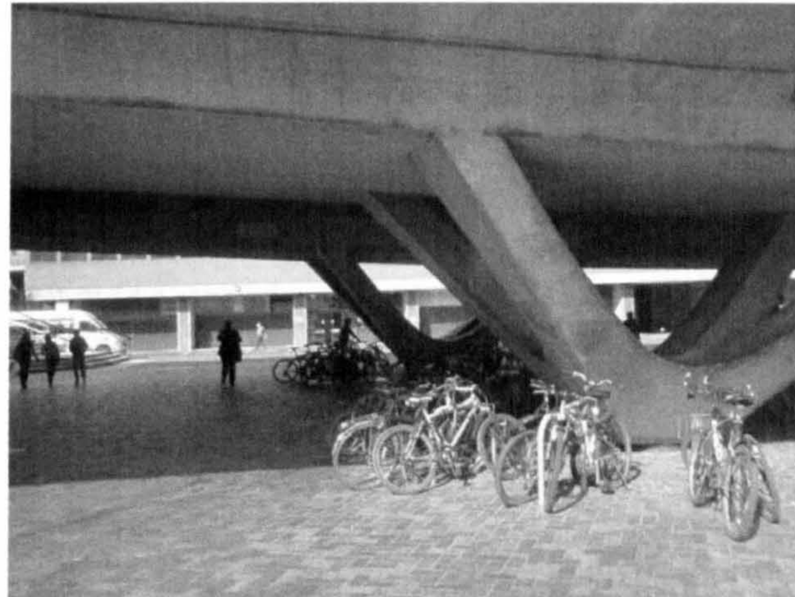
Figure 49: Bike racks under the concourse bridge at Campus site.
