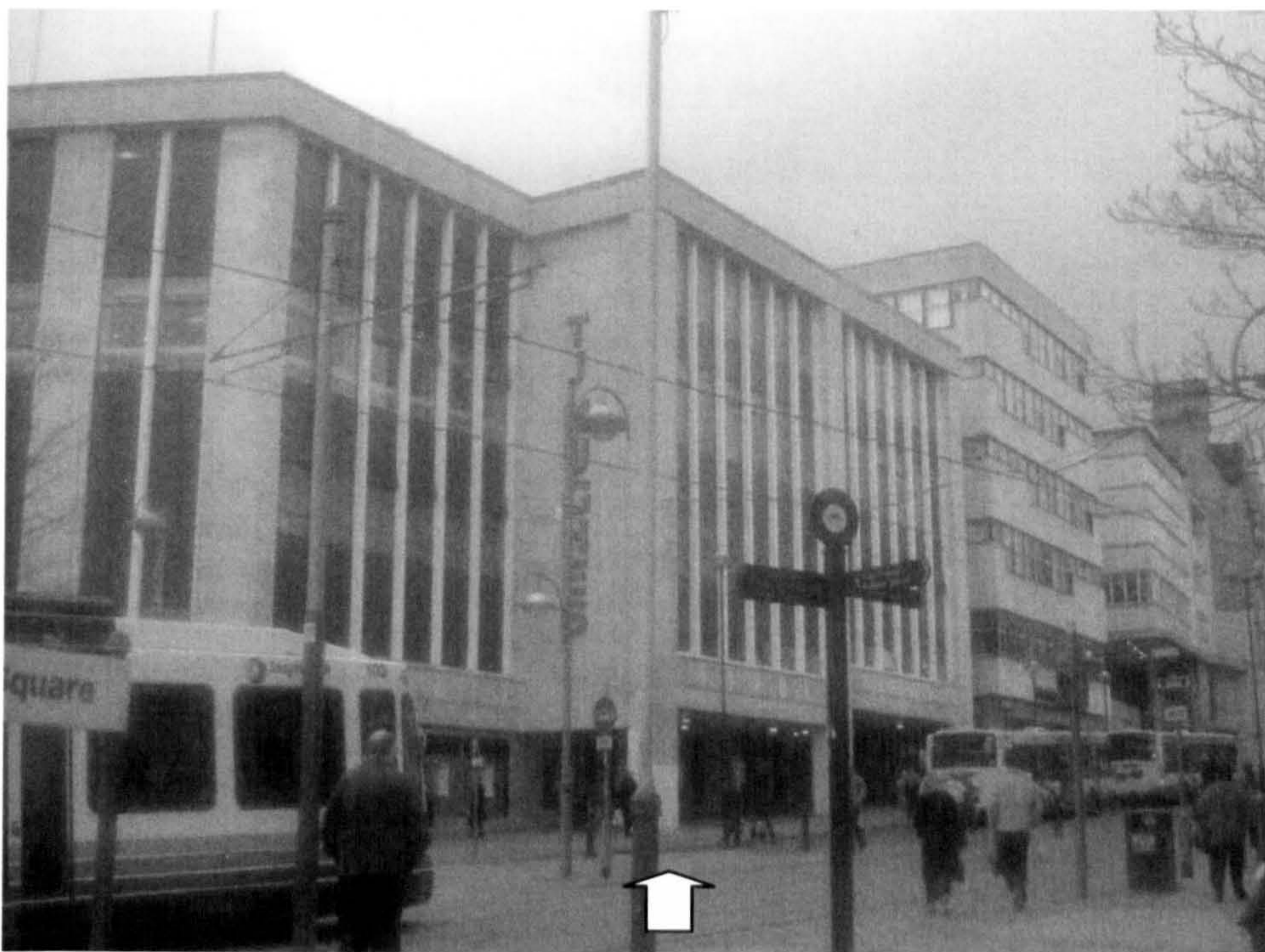
Figure 90: Although not paying any attention to the architectural character of the street, this building in the High street has adopted the use of porticos in order to create a transition to the exterior.
