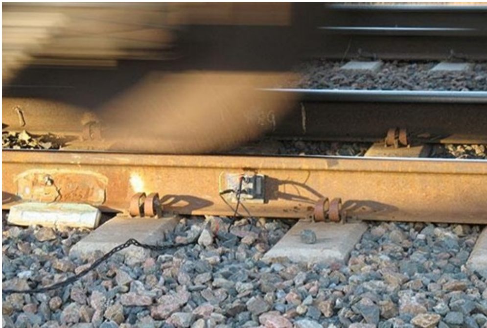
Figure 2.6: An ultrasonic measurement device installed on in-service rail
