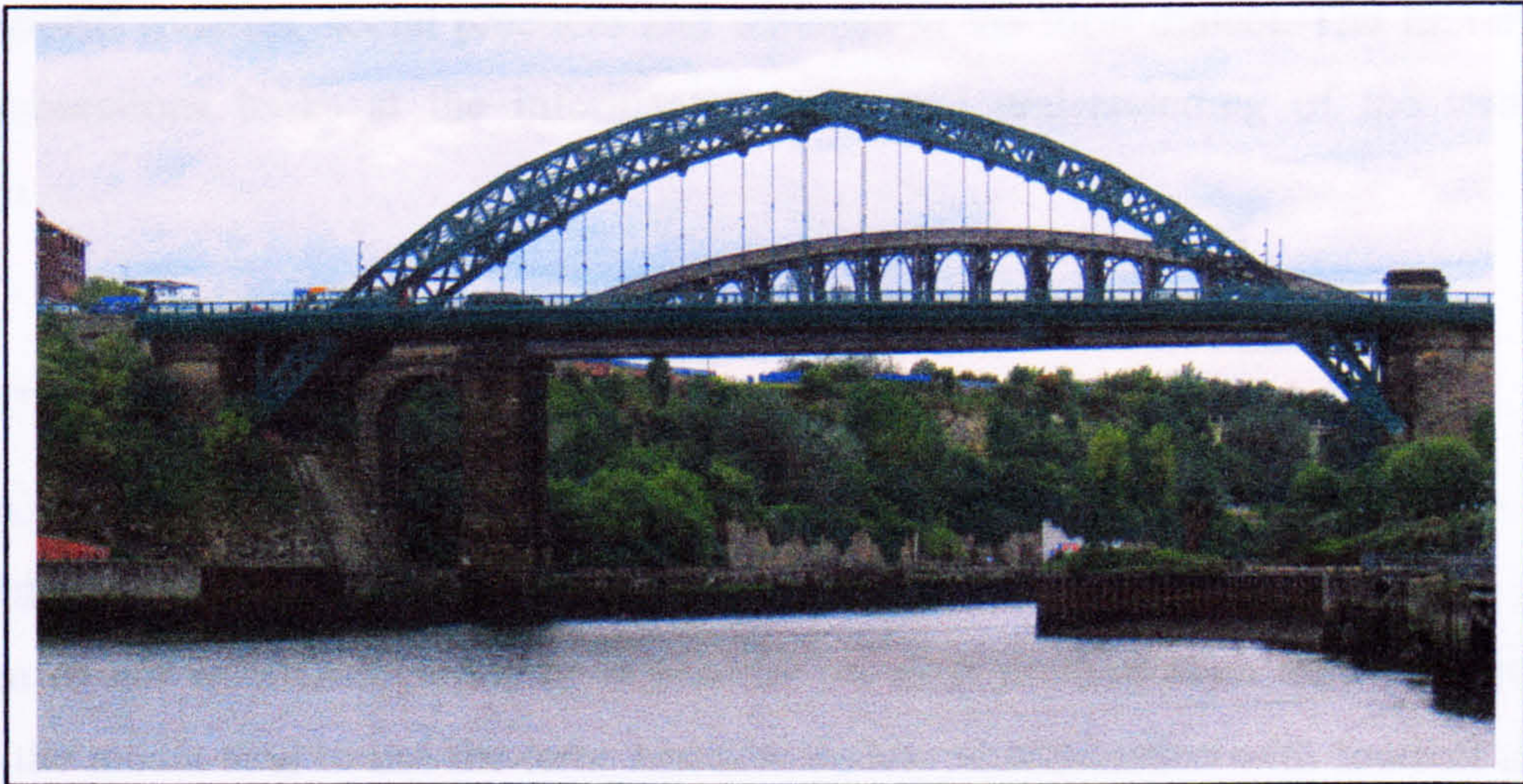
Picture 4.1: Wearmouth Bridge 9
