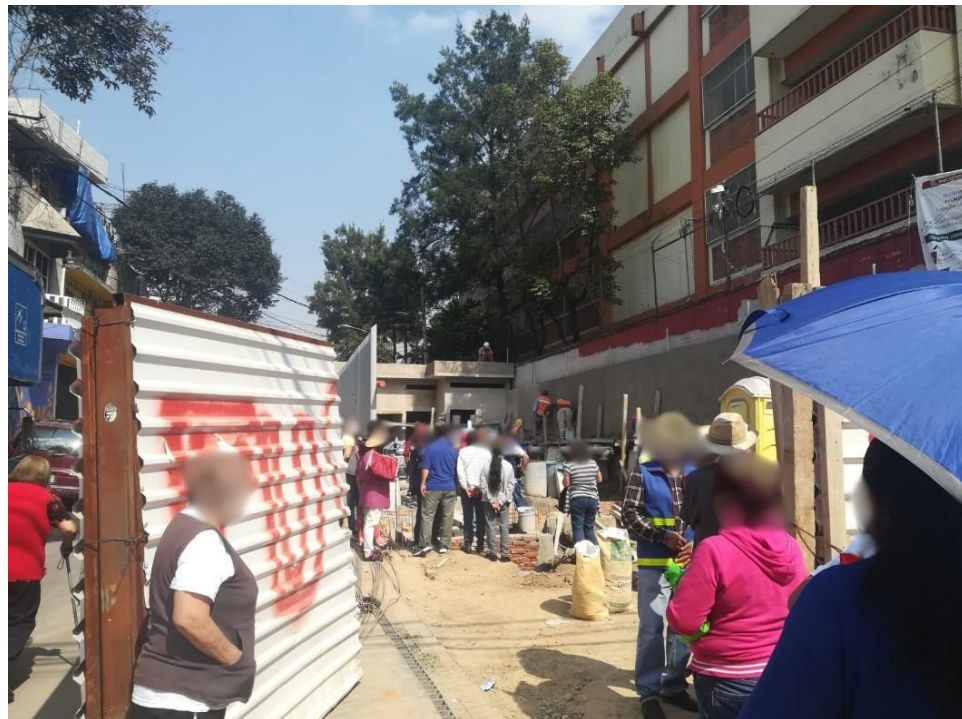
Figure 31. Neighbours entering the construction site Source: taken by researcher 28/11/22
