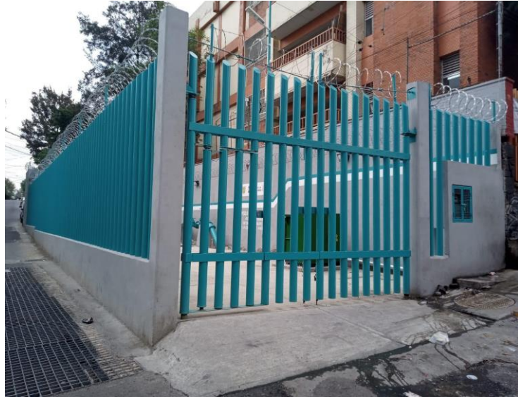
Figure 34. The water well after its completion in 2023 Source: taken by researcher 01/06/23
