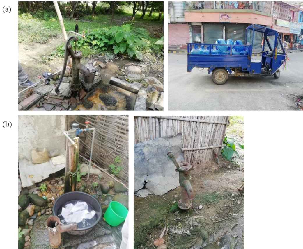
Figure 7.25: Examples of (a) Other Sources of Water Used by Households in Lahan and (b) Non-functioning Tube Wells
