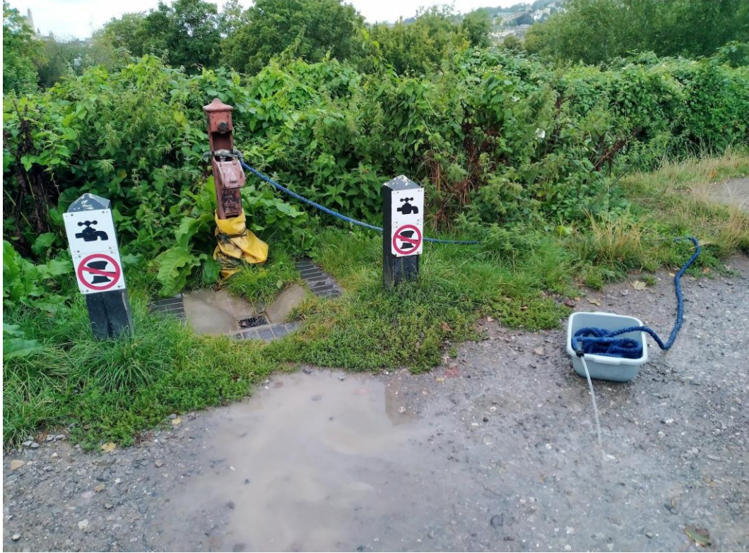
Figure 20: Water provision on the visitor moorings in Bath (Kennet and Avon Canal).
