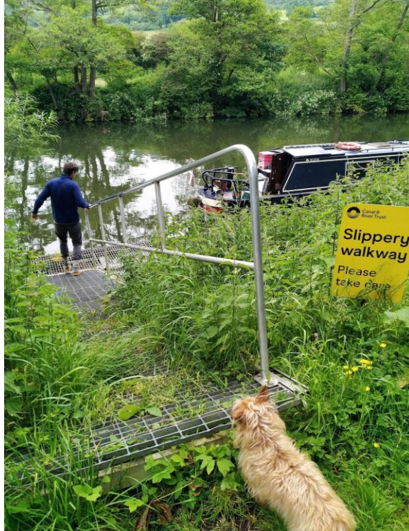
Figure 16: Service station provided by Wessex Water/CRT on the River Avon near Swineford.
