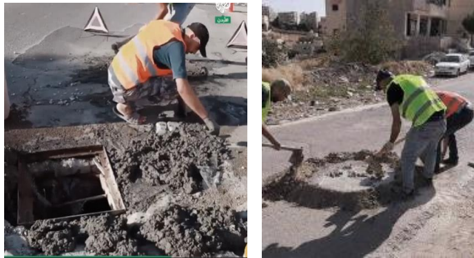
Figure 7.19: Volunteers from Bader Initiative working on fixing a road in Zarqa. Source: ‘Bader’ Initiative, 2021
