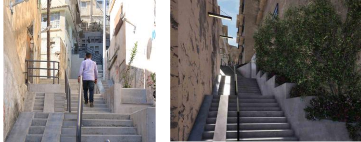
Figure 6.13: Staircase No.7 after GIZ's intervention. Left: The walls at the staircase entrance seem freshly painted and in good condition. Right: This picture was taken at the top of the staircase, where the walls are not fixed or painted. Source: GIZ, 2020
