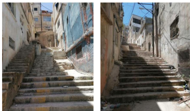
Figure 6.2: Staircase NO.7 condition before the renovation by the GIZ. Source: GIZ, 2019
