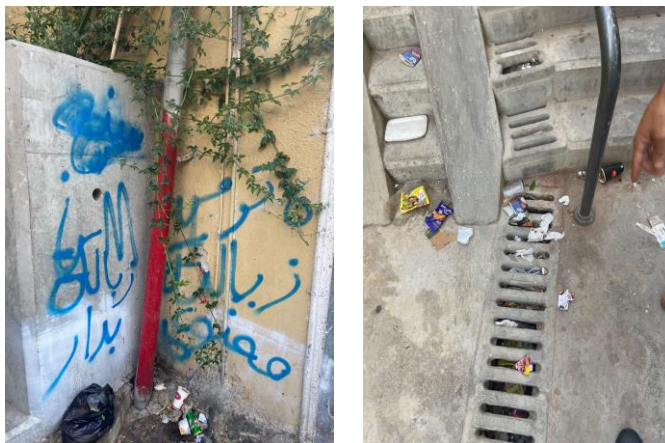
Figure 6.21: The current conditions of the staircase NO.7 site. Author, 2022
