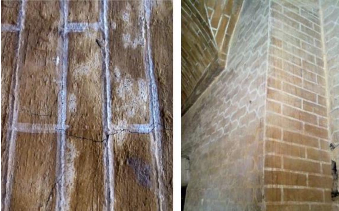
Figure 117: Two views of the painted Ajornama decorations (simulated with painted designs on plaster), Mozaffari Madrassa, Jameh mosque of Isfahan (Author).
