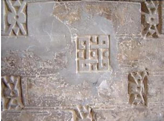
Figure 122: The stucco brickwork 'stamped Ajornama' technique, Jameh mosque of Yazd, Ilkanid period (Author).
