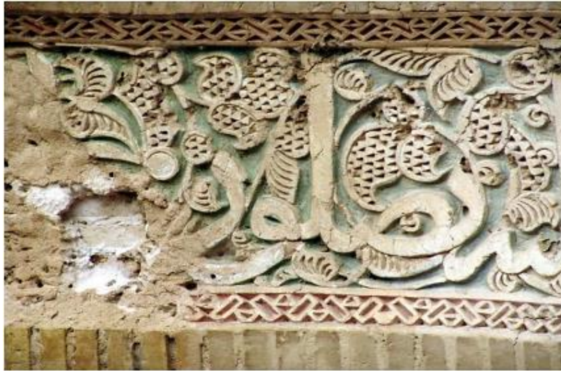
Figure 47: In these decorations, there is a distinctive difference in the level of primary ornaments with their background. The Boomnama relief elaborated stucco ornaments which are in binary (flat and shallow both) technique, the northern Ivan of Jameh mosque, Oshtorjan (Author).
