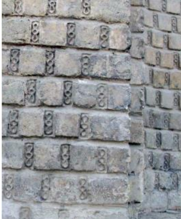
Figure 17: One of the in-situ mold methods in stucco art is the Mohri method which can be seen in Ilkanid stucco carving, in this method the repeating patterns are executed on the plaster layer using a single template. The Mohri patterns were executed in situ using a molding technique, Jameh mosque of Isfahan, attributed to the Seljuk period (Author).
