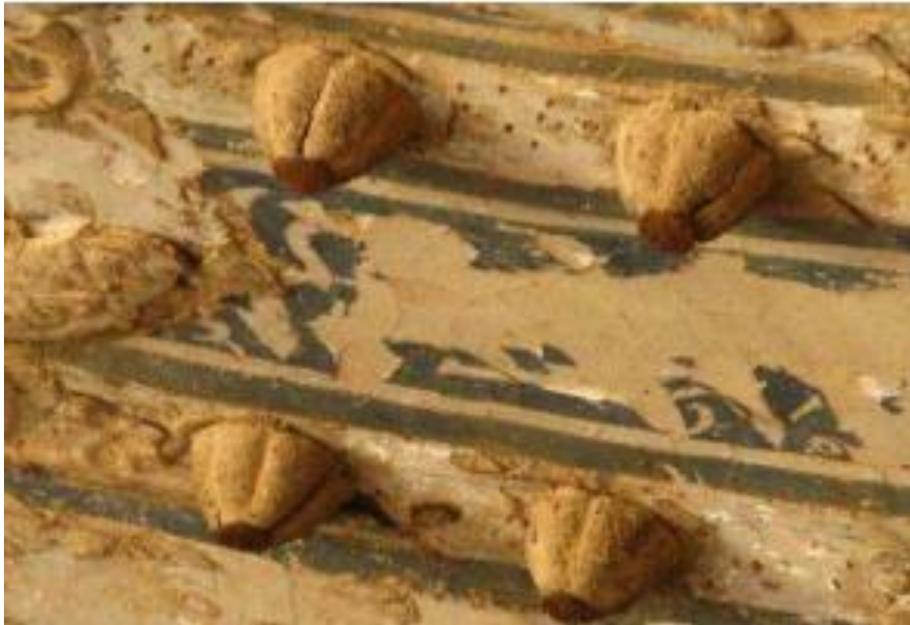
Figure 16: The 'appliqué' method is a method of stucco decorations which is done by adhering or attaching pieces or decorations onto another surface. The appliqué technique is used to affix elements of an ornamentation or structure onto other surfaces, typically using gypsum, ceramics, or other materials. Floral stucco studs executed in an applique method, Shamsiyeh Madrassa, Ilkanid period, Yazd (Author).
