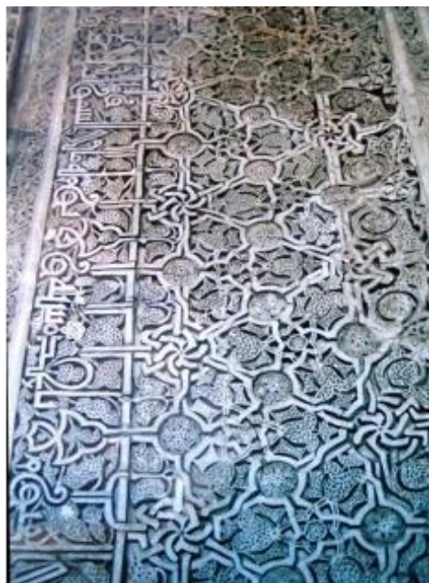
Figure 42: The part of elaborately carved relief Boomnama stucco working with a hollowed background, from the side margin of the Mihrab in the Jameh mosque of Urmia, dating back to the Ilkanid period (Author).
