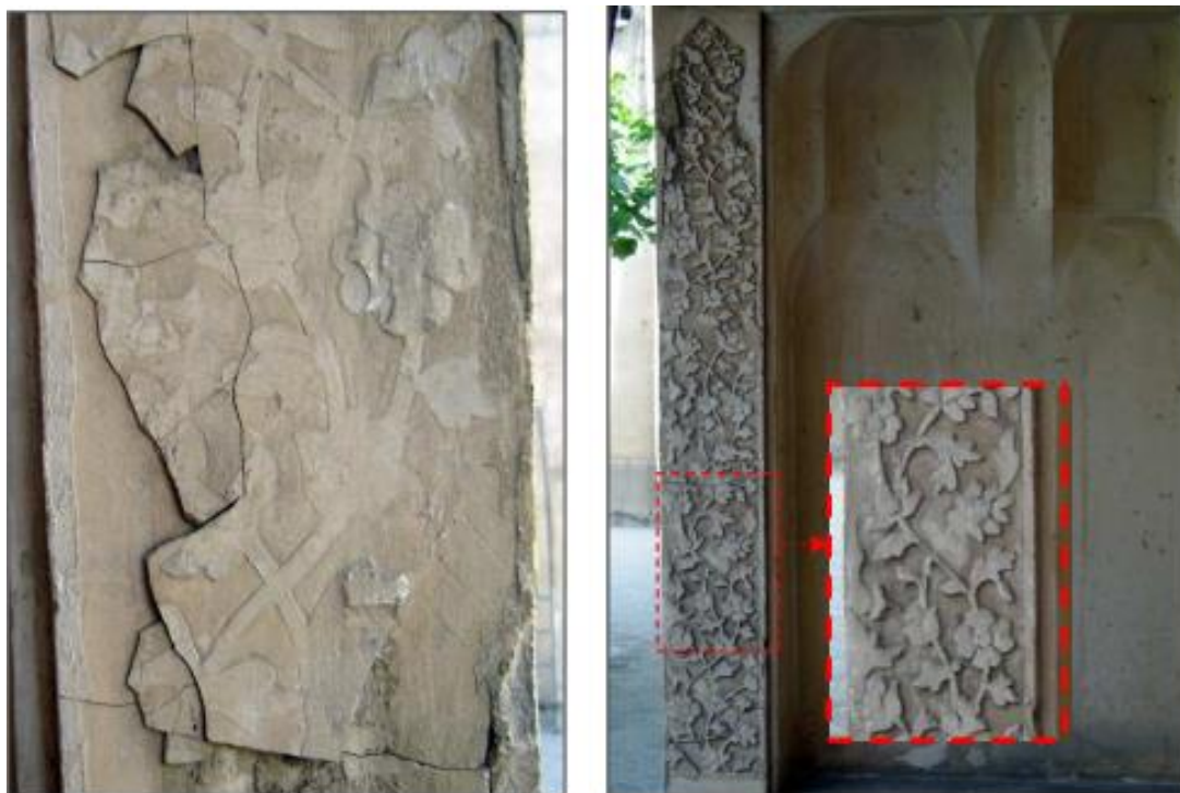
Figure 106: Two views showcasing the low-relief Koshtebori stucco decorations and areas affected by deterioration at the Akhavan-Haghani house in Isfahan, attributed to the Zand-Qajar period (Author).
