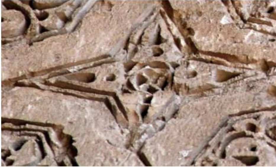
Figure 91: The close-up views depict the surface distortions and the shape deformities of the carved edges, which are part of the prominent gypsum decorations of the Jameh mosque of Farumad in Sabzevar (Borumand 2023).
