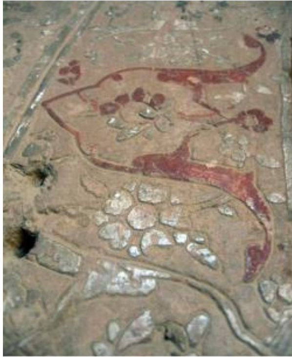
Figure 113: Boom-Saab' stucco with deep groove carvings around the patterns, adorn the Safavid-period Jameh mosque in Isfahan (Author).
