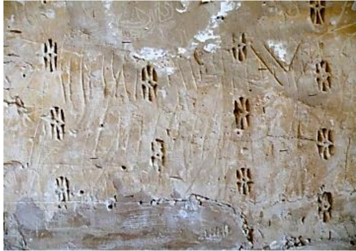
Figure 124: The stucco brickwork 'stamped Ajornama' technique, Jameh mosque of Ardestan, Ilkanid period (Author).
