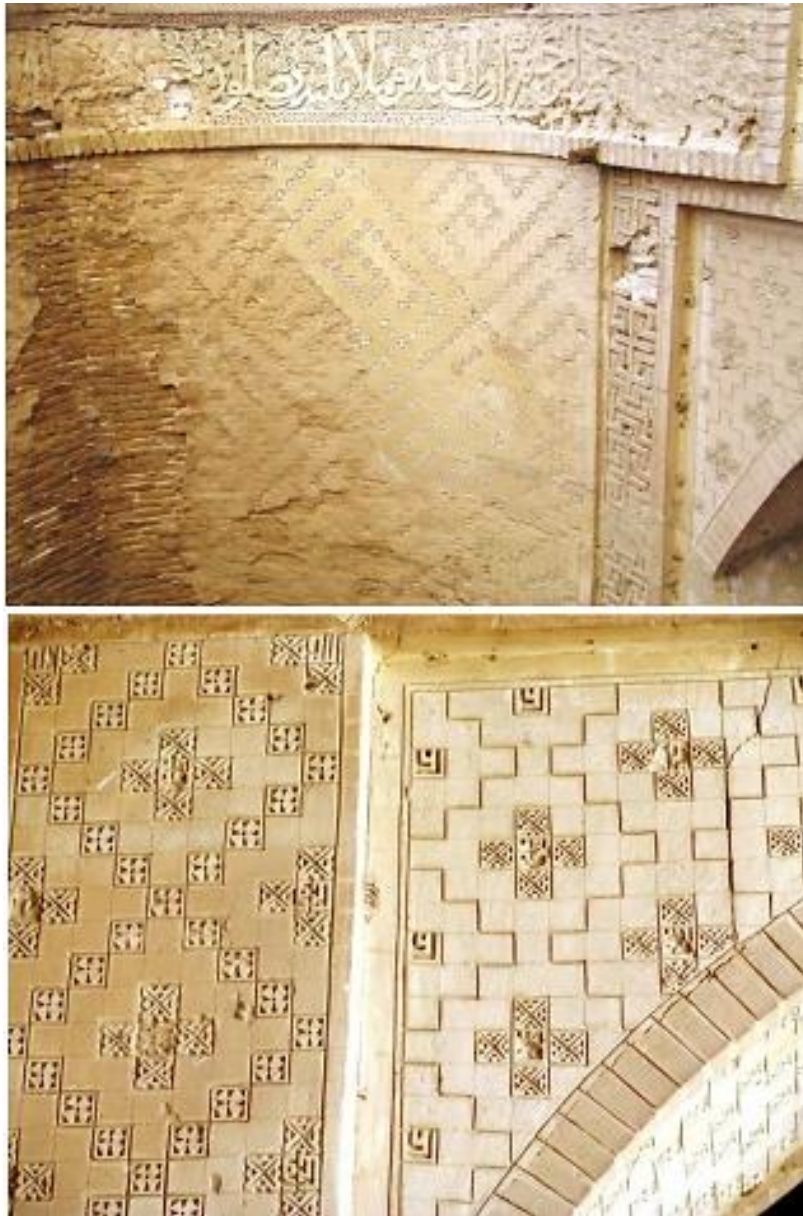
Figure 129: In most Ajornama stucco arrays, the colors used include two dominant hues: Mustard yellow to simulate bricks and white for areas intended to represent gypsum facades. However, other colors such as red, green, blue, and black can also be employed. Two views of the plaster brickwork decorations, remnants of white and mustard yellow paint on the adornments, Jameh mosque of Oshtorjan, Ilkanid period (Author).
