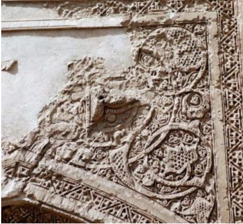
Figure 8: Relief stucco decorations at Farumad Great Mosque, Ilkanid period, Iran. These decorations have less difference in elevation between the motifs and the background. Their intricate patterns and exquisite artistry in this decoration, with a variance in prominence between the stucco's background and the depicted figures ranging from 1.5 cm to 3 cm, justify their categorization as relief stucco (Aslani 2023).
