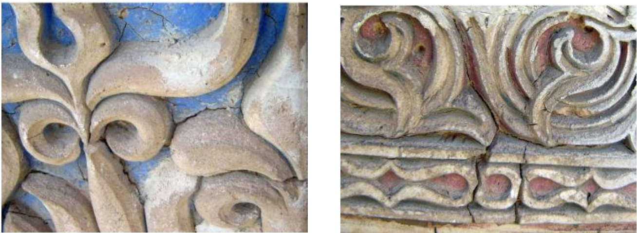
Figure 34: The colorful ornaments were created with the mixture of pigments in the stage of stucco working, especially in the base-coat layer. A close-up view of the elaborate stucco decorations with additional cutting and carving along the edges of the patterns using an inclined method is evident in the decorative border of the Rascat tower in Mazandaran.
