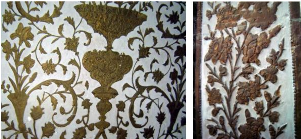
Figure 78: The artist abstains from employing additional colors in the decoration, placing primary emphasis on raised designs and gilding on the white surface. The ‘wood carved-like’ stucco in Ajdehkari technique, which adorned with gold leaf, Seyyed-Shafti Shrine, Seyyed, Isfahan, Qajar period (Author).
