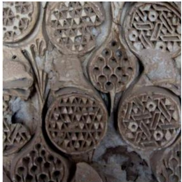
Fig 69: Ajdehkari, duplicative stucco technique, in a hole and geometric method, part of Mihrab of Pamanar mosque, Zavareh, attributed to the Seljuk period (Author).
