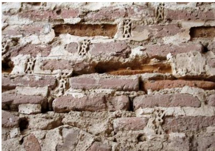
Figure 121: The stucco brickwork 'stamped Ajornama' technique, Ardebil Jameh mosque, decorations dating back to the Ilkanid period (Author).
