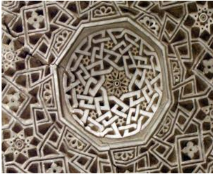
Figure 41: The section of elaborately carved relief Boomnama stucco working with a hollowed background, from the northern Ivan of the Jameh mosque of Isfahan, dating back to the Ilkanid period (Boroumand 2023).
