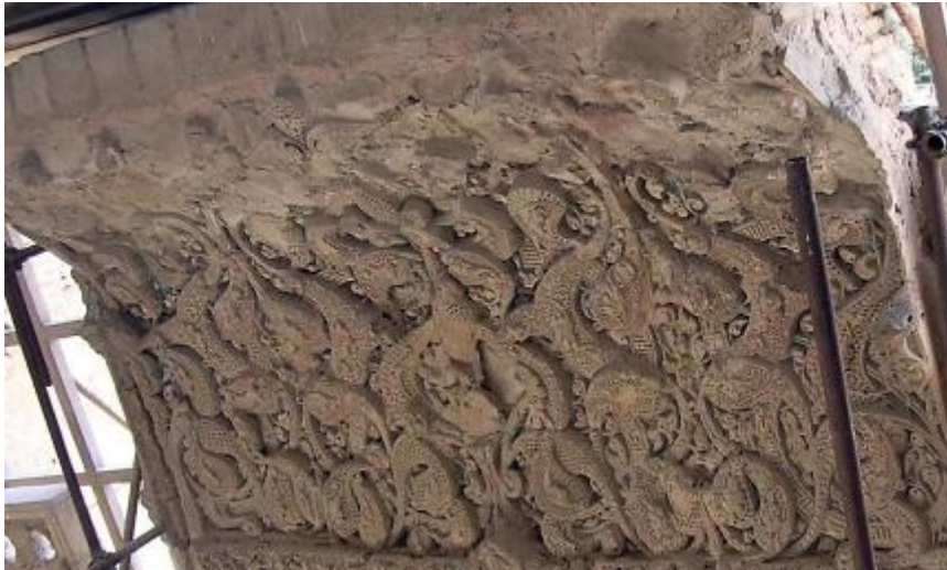
Figure 63: The relief and elaborate stucco decorations in Boomnama ornaments which have been executed in a stratified 'Do-Gacheh' method, the top part of Mihrab's Pir-Bakran shrine (Author).
