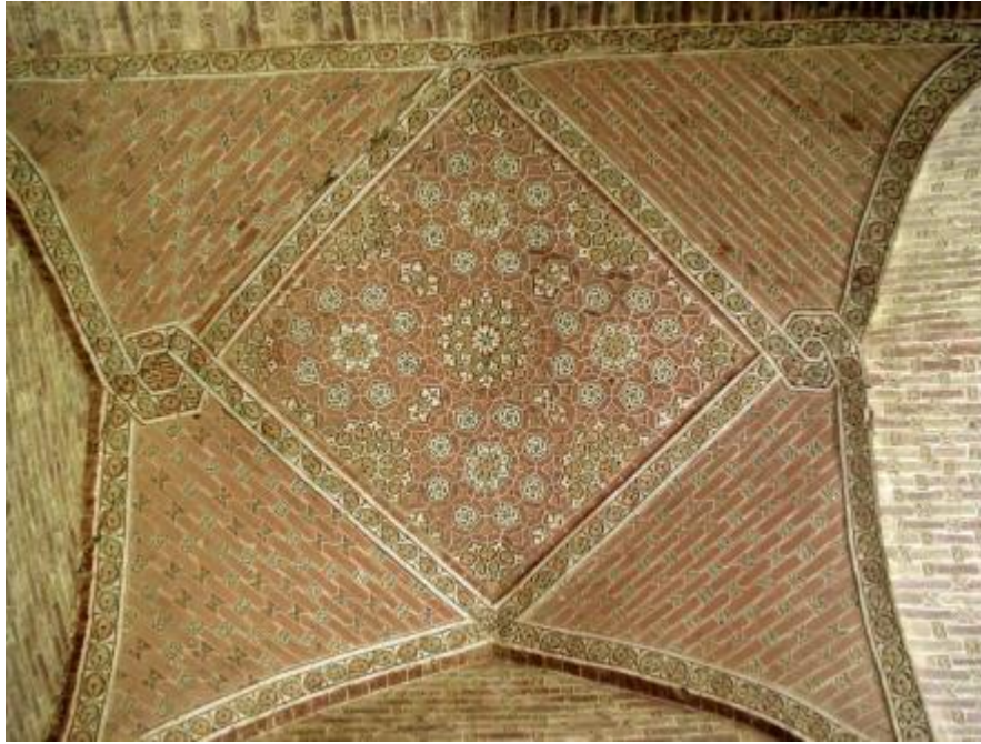
Figure 116: An illustration of the plaster decorations of the Ajornama (simulating low-relief plasterwork with spherical elements and brickwork knots), Sultanieh dome, Zanjan, Ilkanid period (Author).
