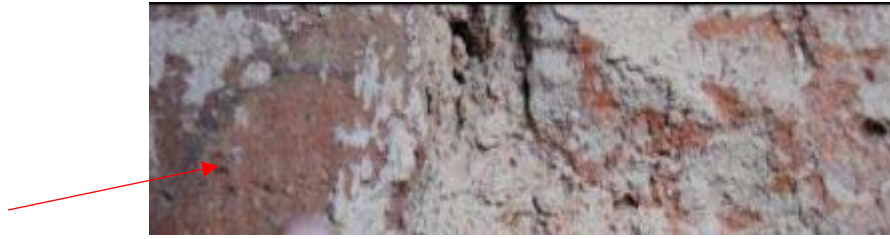
Figure 29: plaster coats used in the underlying layers of stucco decorations confirm the presence of various impurities in the plaster coat mortar. Plaster coat decoration in the vicinity of the Mihrab of the Jameh mosque of Ardebil (Author).
