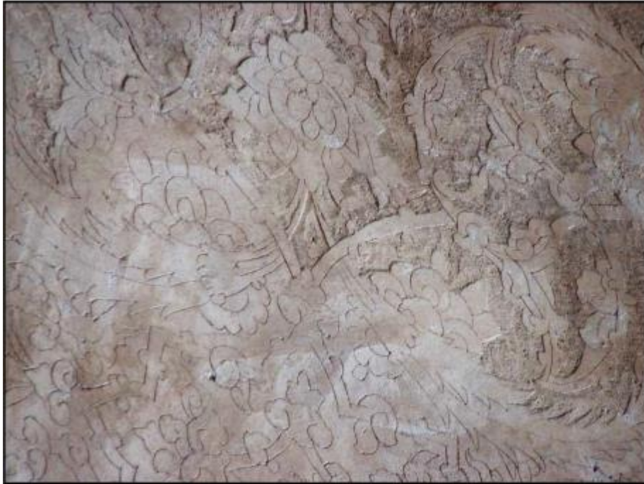
Figure 108: The notable differences in color, texture, and surface between the two layers (basecoat and surface layer) present a significant hypothesis suggesting that the decorations employed in Ali-Qapu might not be Koshtebori decorations.
