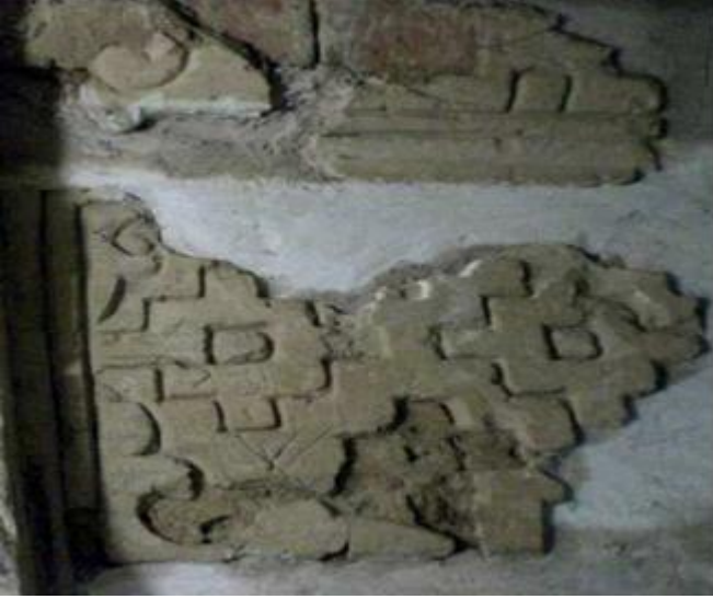
Figure 30: The remnants of simple relief stucco designs, flat cuts, executed by incising lines around the pattern, Jameh mosque of Gonabad (Author).
