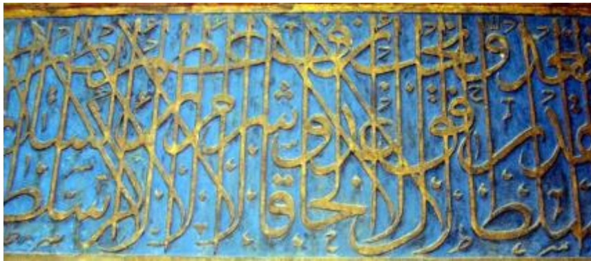
Figure 36: The wonderful sophisticated polychrome ornaments had been created in a Boomnama method, with the color in both the base coat and the plaster coat. Elaborate relief stucco ornamentation, Emamzadeh Ahmad, Isfahan, Qajar period (Author).
