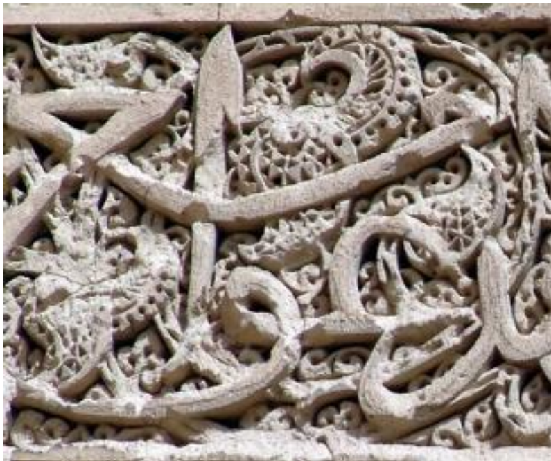
Figure 55: Part of the relief and elaborate stucco decorations in Boomnama ornaments which have been executed in a stratified 'Single-coat- stucco' method, Ilkhanid decorations of Jameh mosque in Oshtorjan (Author).
