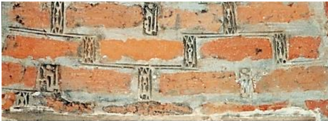
Figure 125: Plaster brickwork 'stamped Ajornama' technique, Jameh mosque of Maragheh Ilkhanid period (Author).
