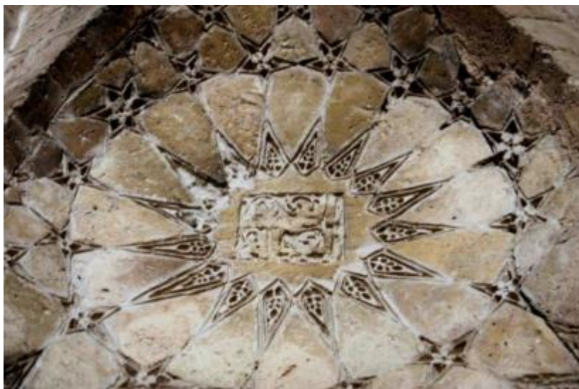
Figure 118: An example of combined Ajornama and stucco decorations, Barsian Jameh mosque, Seljuk period (Author).
