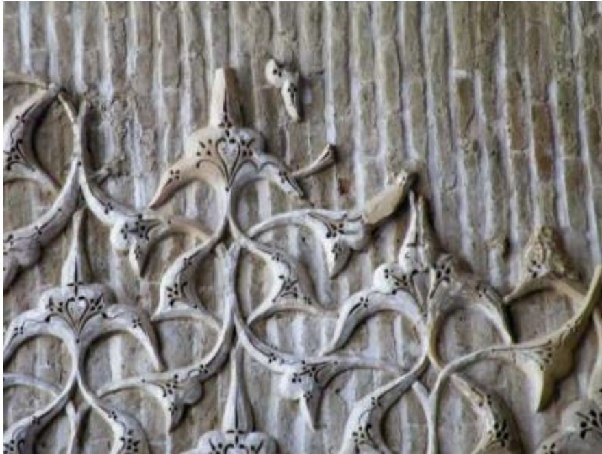
Figure 9: The High-relief stucco decorations with the difference in prominence between the stucco's background and the depicted figures range from 1.5 cm to 3 cm mosque of Ardestan, attributed to the Seljuk period, Isfahan, Iran (Aslani 2023).
