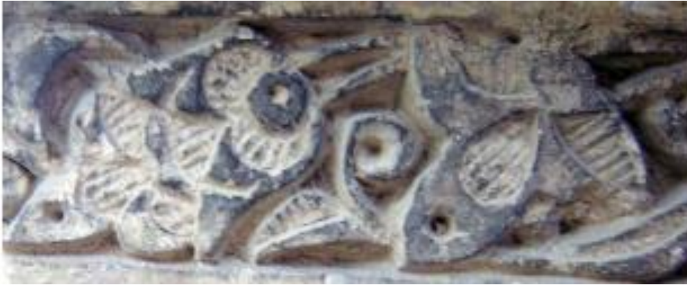
Figure 66: Ajdehkari, is the relief stucco decorations featuring simple scratching that involves texturing the surface of the patterns or texts using straightforward operations like engraving or perforation. The close-up view of the intricate stucco, Ajdehkari, in the scratch style, can be observed in the Jameh mosque of Isfahan, dating back to the Ilkanid period (Author).
