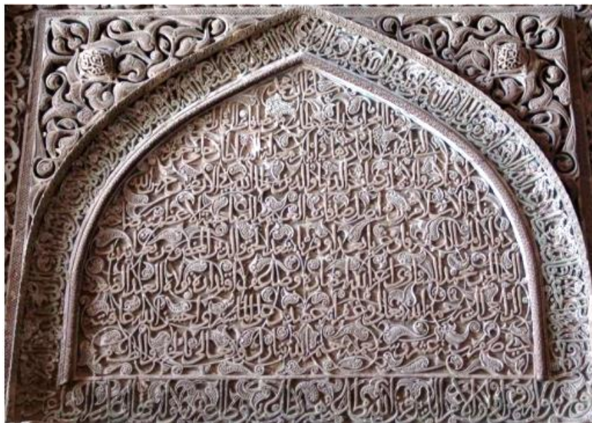
Figure 51: The relief elaborate Boomnama stucco in a dual (plain and patterned) flat style with small lace-like patterns, in the middle section of the Mihrab of Oljaytu's mosque in Isfahan, dating back to the Ilkanid period (Author).
