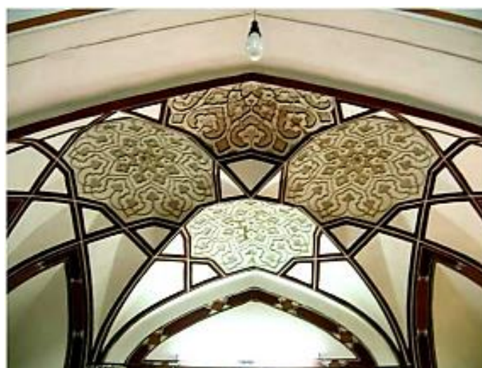
Figure 112: The stucco decorations in the indigenous 'Boom-Saab' style refer to the carved patterns on plasterwork instead of a plain background, in Sharbat-Khanah of Qeisariyeh transom, Isfahan, Safavid period (Author).
