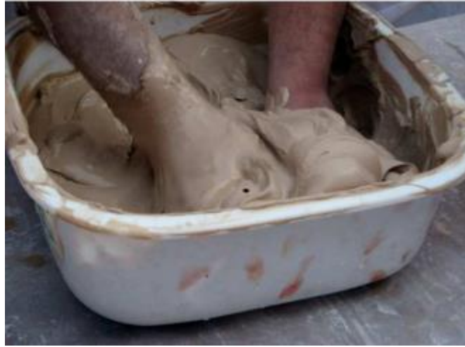
Figure 94: To make pure gypsum plaster in this stucco technique, 65% to 85% water by weight is added to the gypsum. The terms 'kneading' and 'beating' refer to the process of working the mixture of gypsum and water to prepare incised gypsum or Gach-e-Koshteh for the Koshtebori technique (Author).
