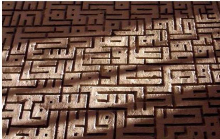
Figure 35: The ‘continuous’ which is named ‘Peivasteh’ stucco decoration, where patterns are densely arranged together. Elaborate and continuous relief stucco ornamentation, Kufic inscriptions on brick structure, Pir-Bakran Shrine, Ilkanid period (Author).
