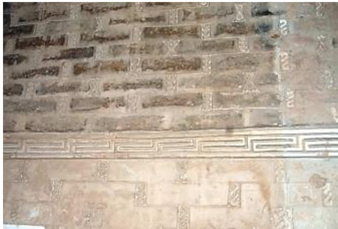
Figure 123: The stucco brickwork 'stamped Ajornama' technique, Jameh mosque of Saveh, Ilkanid period (Author).
