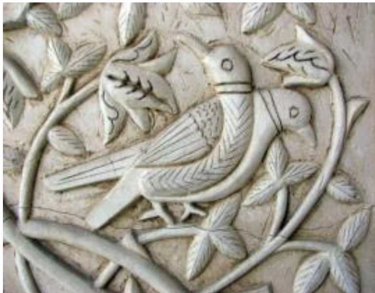
Figure 67: The stucco decorations of the simple Ajdehkari technique through deep incisions on the surface of the patterns. The close-up view of the intricate stucco, Ajdehkari in the 'scratch-style, Kolehdooz house, Yazd, Qajar period (Author).
