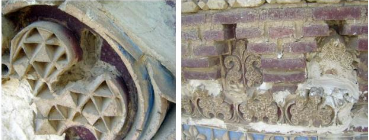
Figure 68: The colorful sections of these decorations were primarily situated in the background, while the carved sections, due to the use of scratching and decoration on the surface of the stucco layer, remained raw and devoid of color. Ajdehkari ornaments, beneath the dome of Rasakht Tower, Mazandaran, attributed to the Ilkanid period (Author).
