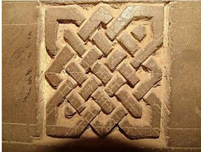
Figure 127: A close-up view of the tool marks of cutting and carving, the grooves related to the grid pattern of low-relief plasterwork mimicking rounded brick bottoms, Grand Jameh mosque of Yazd, attributed to the Ilkanid period (Author).
