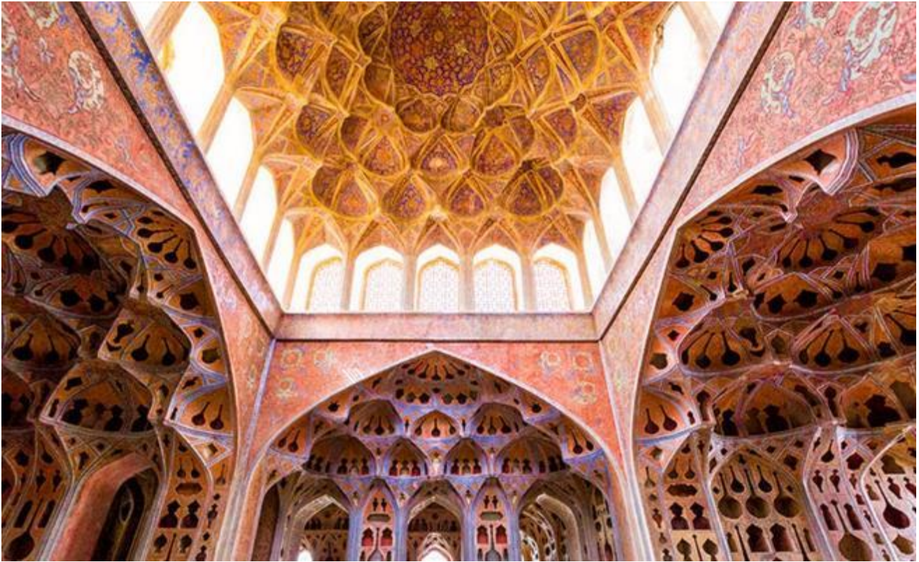
Figure 6: The coexistence of prominent stucco decorations in Ali-Qapu palace in Isfahan, from the Safavid period. These ornaments are known as 'Koshtabri' and 'Tangabri' decorations in traditional Iranian architecture, which are executed in two very different techniques and at completely different levels of projection (Author).
