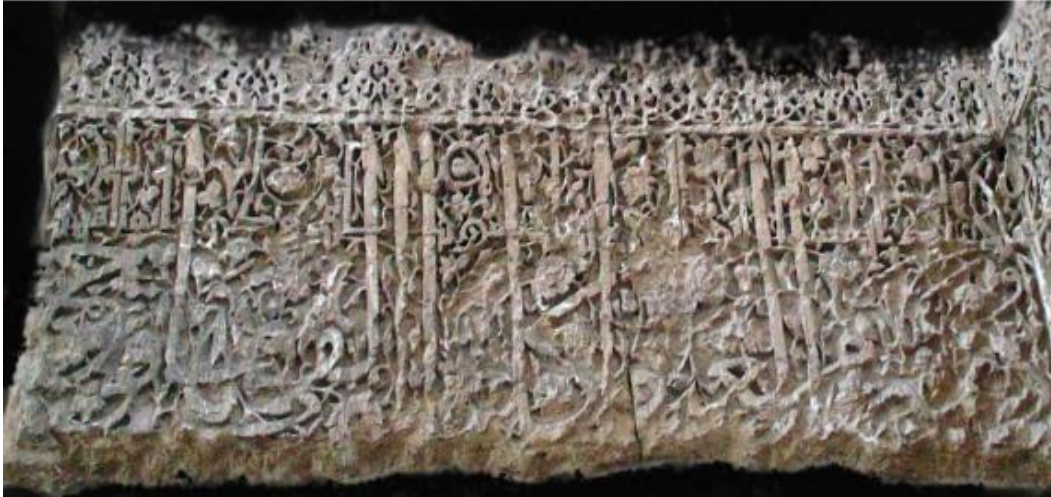
Figure 38: The elaborate Boomnama stucco belonging to the Sultanieh dome in Zanzan. The separation and lines of demarcation observed along the edges of the Boomnama stucco patterns in the decorative margin of this decoration indicate that the gypsum background layer has been applied after the formation of the stucco decorative patterns, in the spaces between the executed patterns (Aslani 2023).
