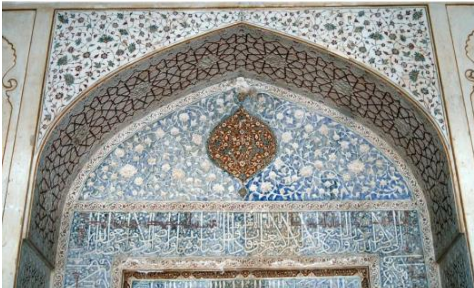
Figure 15: 'Tokhme Gozari' is one of the traditional stucco techniques characterized by various decorative motifs, geometric patterns, and floral designs. These decorative elements are created through engraving and filling with colorful mortar. Stucco is mixed with natural pigments to achieve different colors and applied to surfaces such as walls, ceilings, and architectural features. The Tokhme Gozari stucco work is showcased in the Saveh Great Mosque, dating back to the Safavid period (Author).
