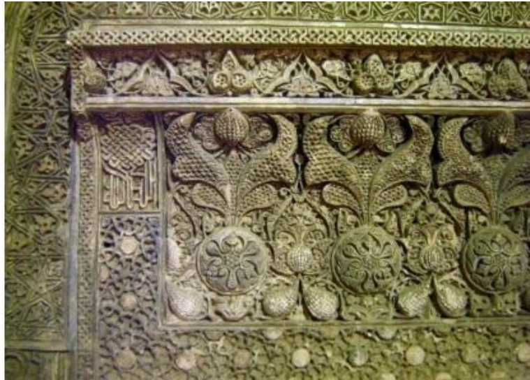
Figure 87: The combined technique of the reliefs stucco with the inclined incised Ajdehkari style and stamped decorations, Mihrab of Jameh mosque, Isfahan, Seljuk period (Author).
