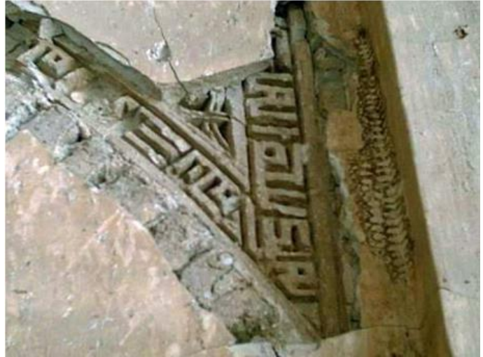
Figure 33: Simple raised gypsum decorations, flat incisions, incised lines around the patterns, Jameh mosque of Saveh, Ilkanid period (Aslani 2023).
