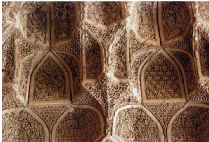
Figure 80: The curving Ajdehkari technique in stucco of the Muqarnas decoration of the Mihrab of Muqarnas, Jameh mosque in Farumad, Sabzevar (Author).
