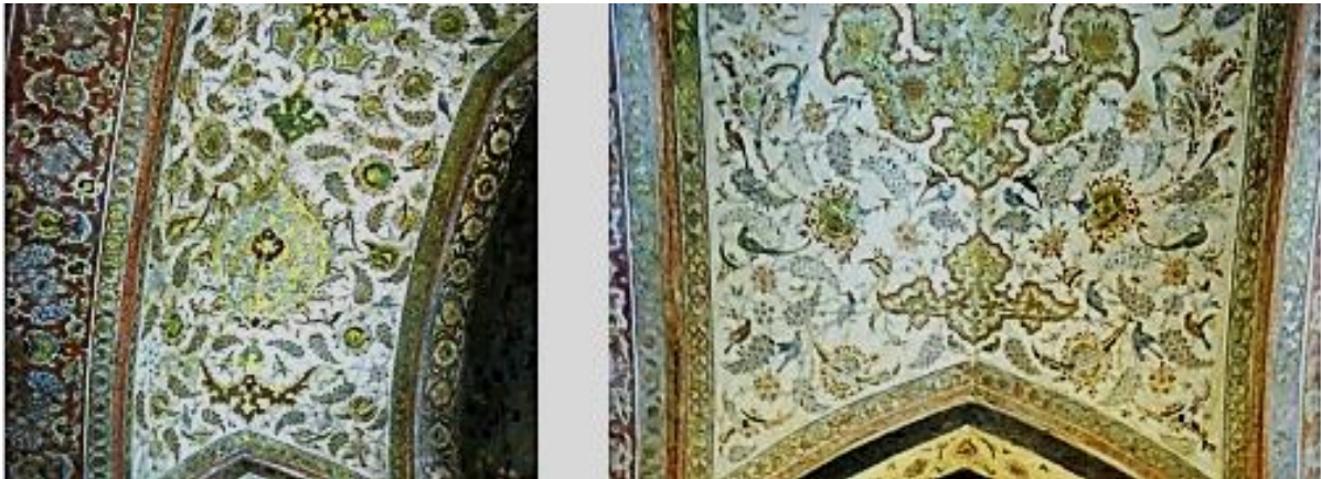
Figure 111: Sections of the Alcoves and Niches in the side rooms of the Chehel-Setoun Palace in Isfahan, adorned with gold leaf decorations, showcased features of Safavid-period subsurface relief decorations. In this technique, the stucco artist meticulously carved relatively deep grooves around the motifs, accentuating their shapes. Two views of indigenous dome-shaped vaults, accompanied by gold ornamentation, from the Safavid period, can be seen in the Chehel-Setoun palace in Isfahan (Author).
