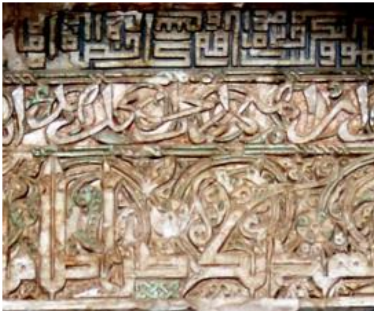
Figure 53: In some stucco decorations, the main patterns and background designs are carved at varying depths into a single surface. This method, in traditional terminology, is called ‘Yek-Gacheh’ or ‘Single-coat- stucco’. Part of the relief and elaborate stucco decorations in Boomnama ornaments have been executed in a stratified ‘Single-coat- stucco’ method, Mihrab Ilkanid of Jameh mosque in Saveh (Borumand 2023).
