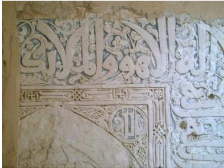
Figure 105: The low-relief stucco decorations, possibly achieved through Koshtebori, adorn one of the tripartite Mihrabs from the Seljuk period in the Saveh mosque (Author).
