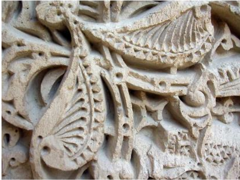
Figure 56: Part of the relief and elaborate stucco decorations in Boomnama ornaments which have been executed in a stratified Single-piece- stucco method, Ilkanid decorations of the lintel and portal spandrel of Pir-Bakran shrine's entrance (Author).
