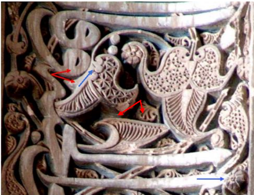
Figure 65: The two sections delineated by red arrows indicate the underlying base layer. One layer comprises the complete background pattern volume in the lowest tier of decorations, while the other underlying layer represents the more prominent raised patterns in the second tier of decorations which are indicated by blue arrows . The relief and elaborate stucco decorations in Boomnama ornaments have been executed in a stratified Se-Gacheh method, the Mihrab of Oljaytu in the Jameh mosque of Isfahan (Author).
