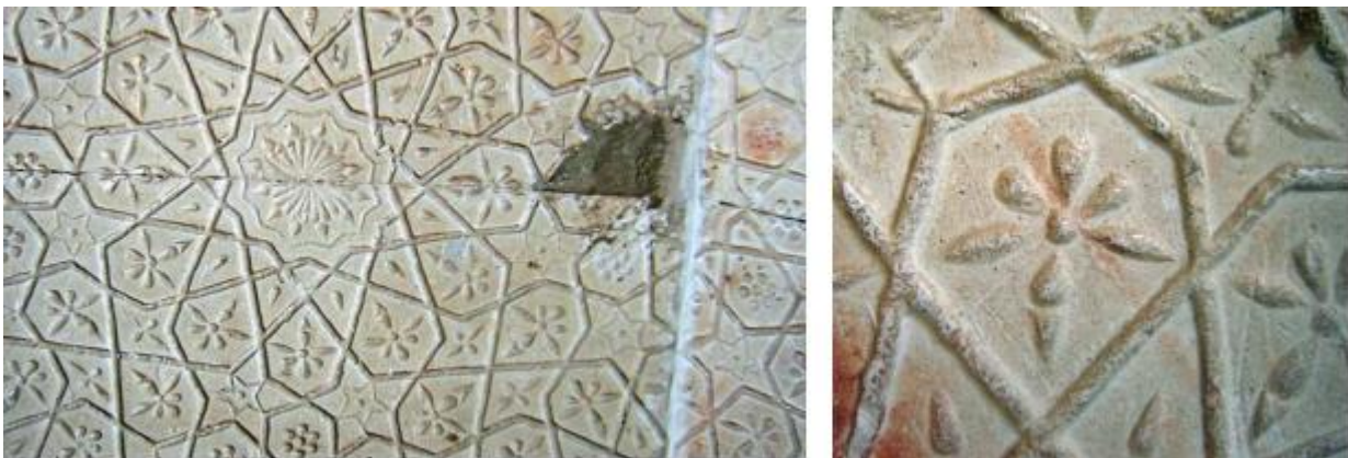
Figure 119: The stucco classified as the Mohri technique is the Ajdekari decorations created through molding techniques with relatively high-relief ornaments. Ajornama decorations (executed using molding technique), Jameh mosque of Gonabad, adornments dating back to the Qajar period (Author).
