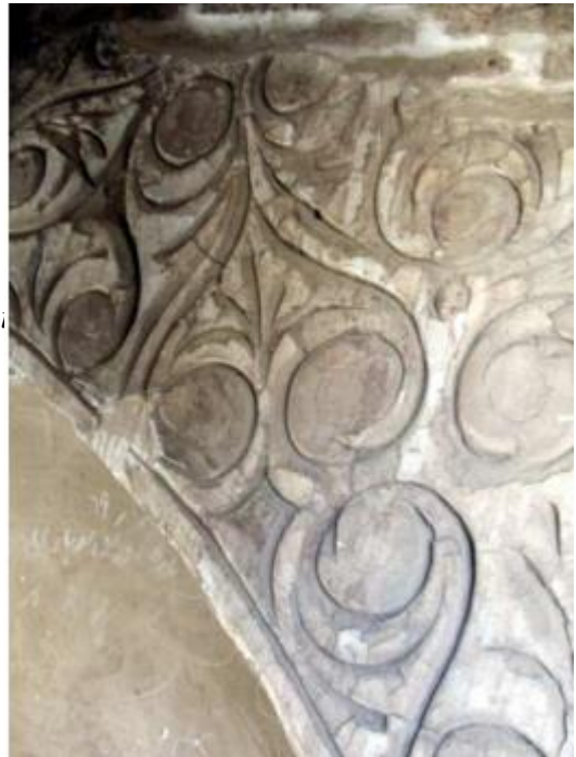
Figure 31: Simple relief stucco decorations in Indigenous style, inclined cut method, Pamemar mosque in Zavareh, Seljuk period (Author).
