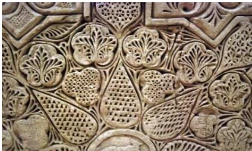
Figure 86: Often, stucco works present an artistic amalgamation of various techniques, a fusion of executed Ajdehkari works using numerous methods such as perforation, carving, incised knotwork, or curved lines. These techniques are realized by employing diverse cutting and carving methods on stucco. The combined technique of the reliefs stucco with the inclined incised Ajdehkari style and stamped decorations, Neishabor Madrassa, 12 th century (Aslani 2011, 68).
