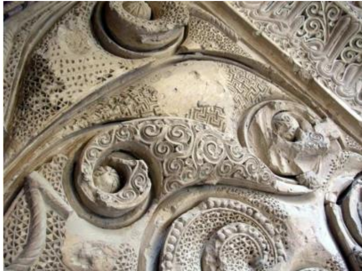
Figure 89: The combined technique of the reliefs stucco with the inclined incised Ajdehkari style and stamped decorations, Mihrab of Pri-Bakran Shrine, Lenjan, Isfahan, Ilkanid period (Author).
