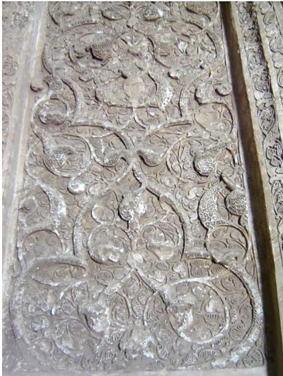
Figure 58: Part of the relief and elaborate stucco decorations in Boomnama ornaments which have been executed in a stratified double-coat-stucco method, Ilkanid decorations, Alavian dome in Hamadan (Author).
