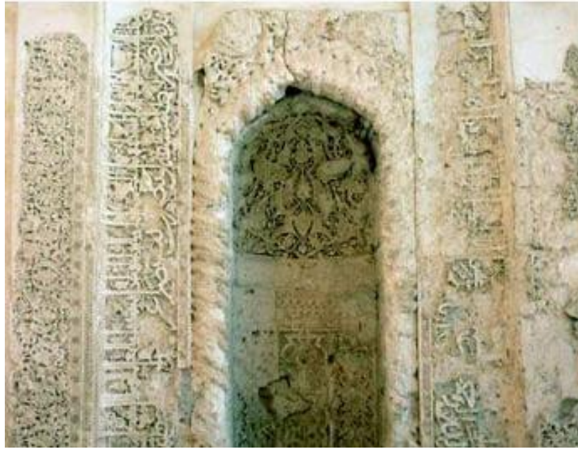
Figure 62: The relief and elaborate stucco decorations in Boomnama ornaments which have been executed in a stratified Do-Gacheh method, the eastern Ivan's Mihrab in Jameh mosque, Abarkooh.in Yazd (Author).
