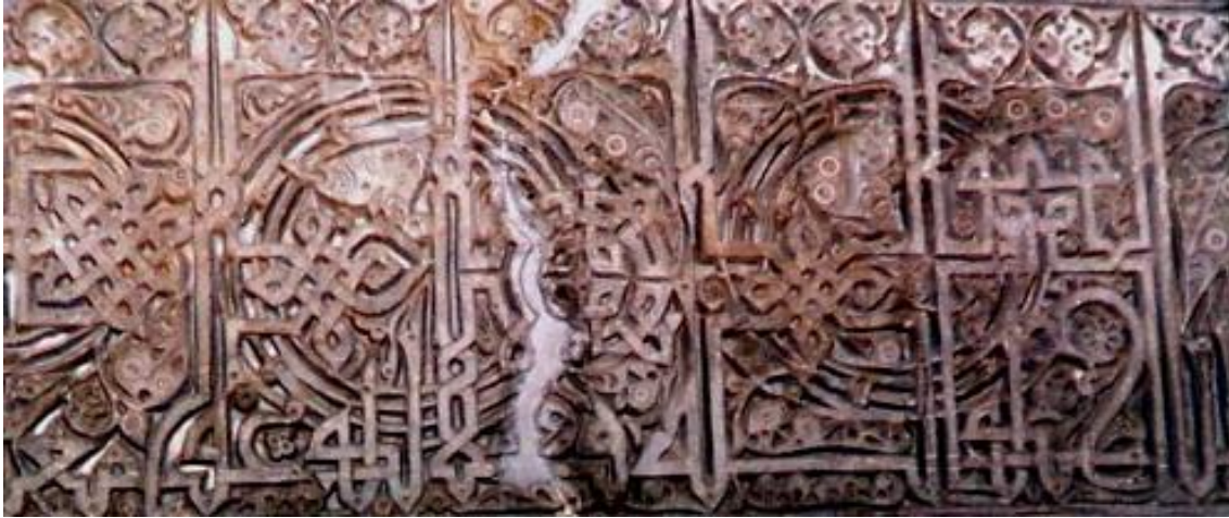
Figure 45: In some stucco decorations there is a distinctive difference in the level of primary ornaments with their background. The relief is Boomnama, elaborated flat ornaments in the stucco working of Bayazid, Bastam's Kufic script inscriptions (Aslani 2023).
