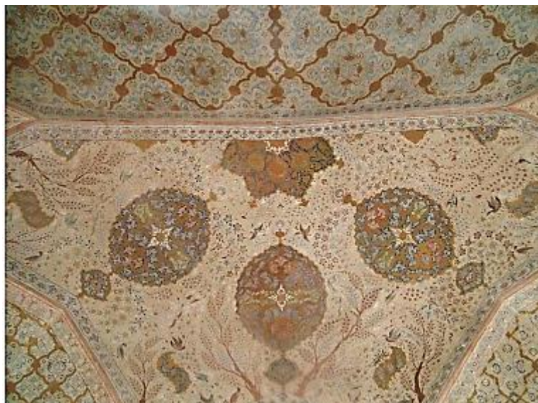
Figure 107: A portion of the subsurface relief stucco decorations of Boom-Saab can be found on the ceiling of the central hall on the third floor of the Ali-Qapu Palace in Isfahan (Author).
