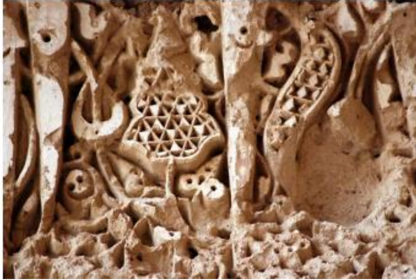
Figure 54: In the Single-coat- stucco decorations, the main patterns and background designs are carved at varying depths into a single surface. Part of the relief inscription in a stratified 'Single-coat- stucco or Yek-Gacheh method of the Mihrab in the Jameh mosque of Farumad, Sabzevar (Peimani 2023).
