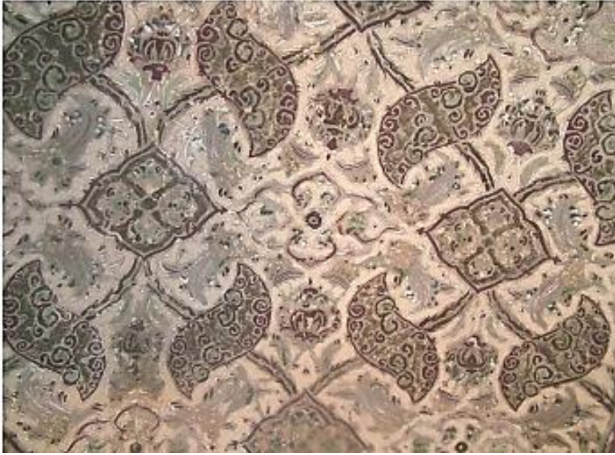
Figure 109: Unlike other buildings with similar-looking decorations, Ali-Qapu exhibits minimal surface disparities, sometimes limited to slight roughening of certain design areas. Moreover, the absence of surface layer separation from the underlying layer in comparison to similar decorations signifies differences in the material properties and execution method between this structure and other comparable samples. The part of the low-relief stucco decorations in Boom-Saab technique, Ali-Qapu Palace, Isfahan, Safavid period (Author).
