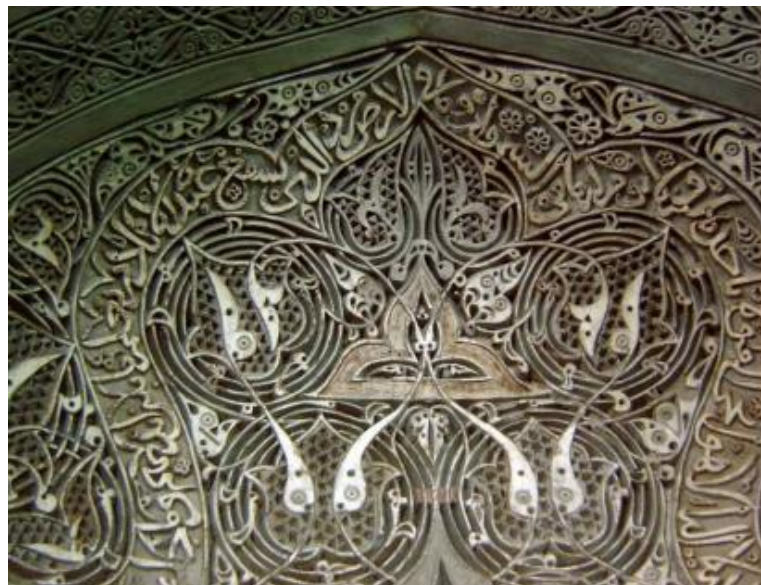
Figure 88: The combined technique of the reliefs stucco with the curved incised and stamped decorations in Ajdehkari style, Bayazid Complex, Bastaam, Ilkanid period (Author).
