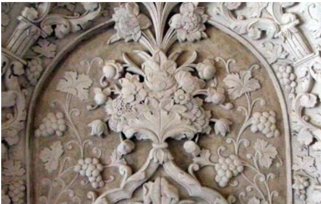
Figure 77: The 'wood carved-like' stucco in the Ajdehkari technique, which had been executed in the Western artistic styles, Colonel Vasigh-Ansari's house, Isfahan, Qajar period (Author).
