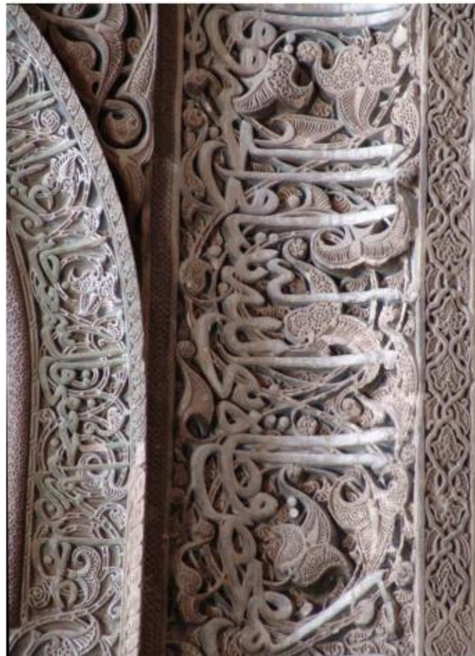
Figure 90: The combined technique of the reliefs stucco with the inclined incised and stamped in Ajdehkari decorations, Mihrab of Jameh mosque, Isfahan, Ilkanid period (Author).
