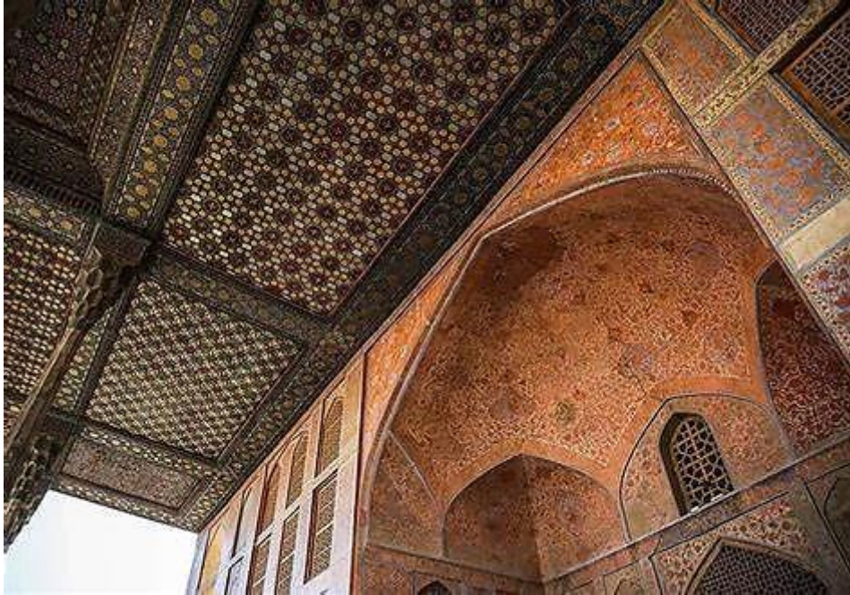
Figure 12: There has been a wide range of stucco works that have been made in a low-relief method. One of the distinctive features of low-relief stucco decorations in the architectural style of the Ivan of Ali-Qapu, Isfahan, during the Safavid period (Boroumand 2023).
