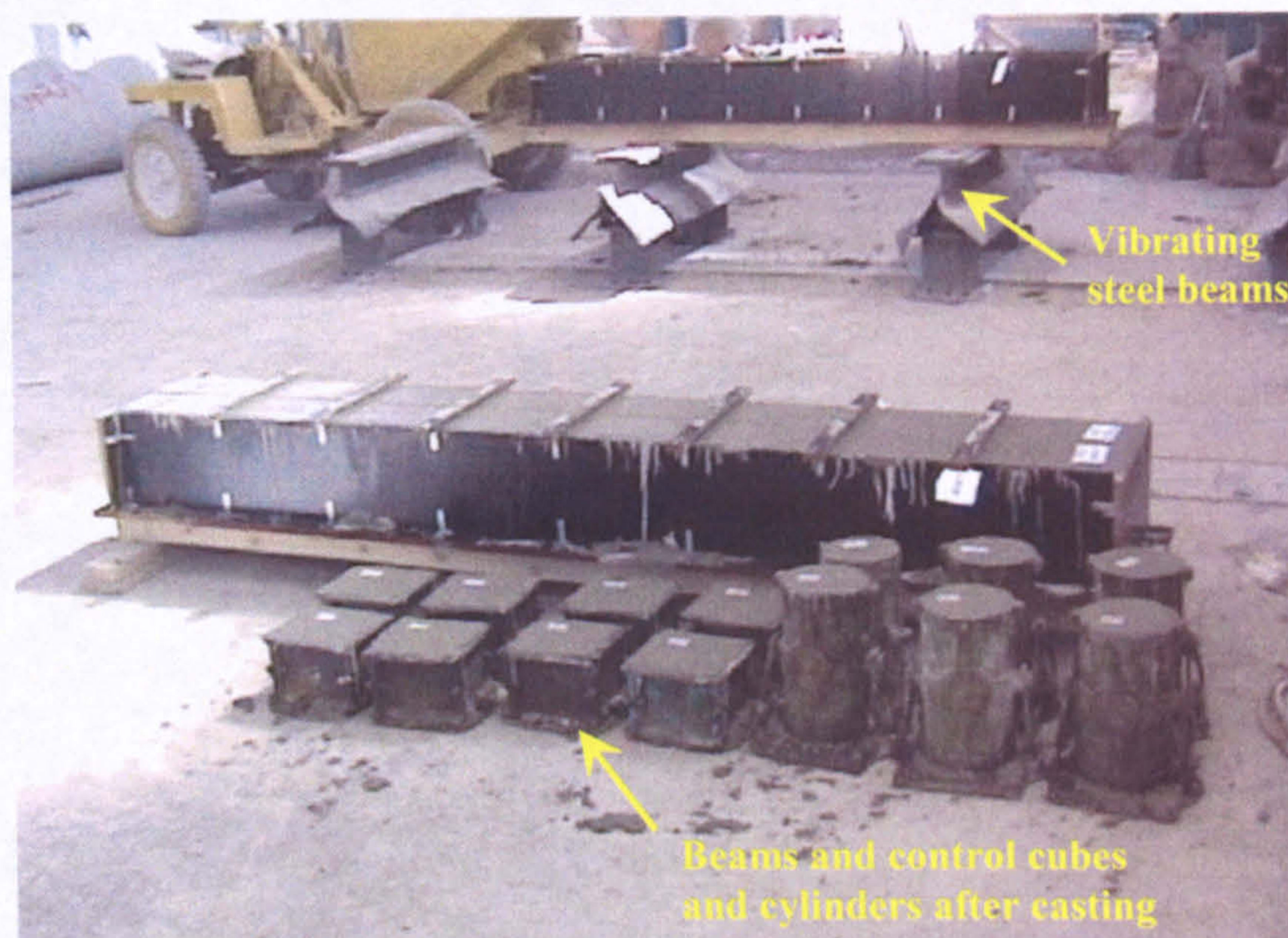
Figure 3-7: Vibrating steel beams used for vibration of concrete.
