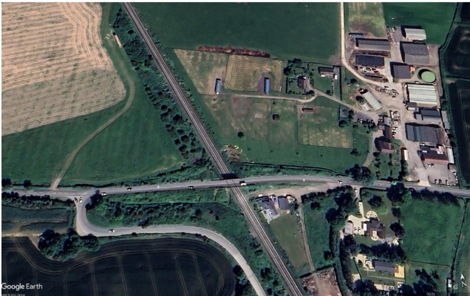
Figure B.3: ©Google Earth 2023 image of the gas leak site taken in June 2023, showing works being done on the west side of the railway line.
